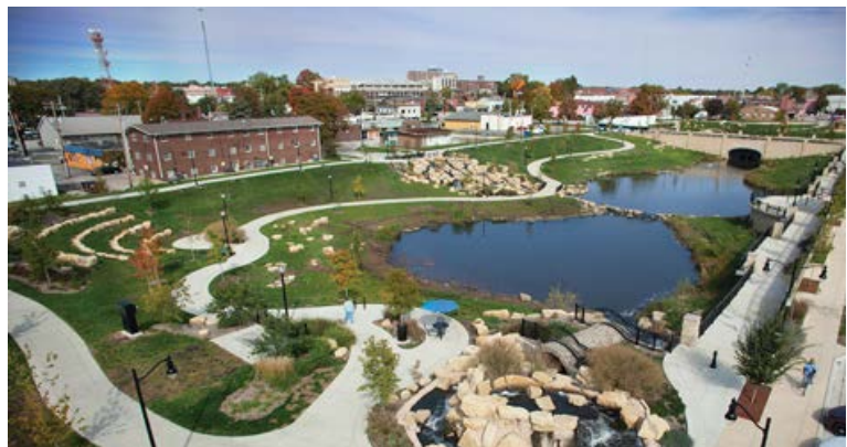
Figure H.4: Regional detention basin in Champaign, IL. Photo courtesy of FOTH.
