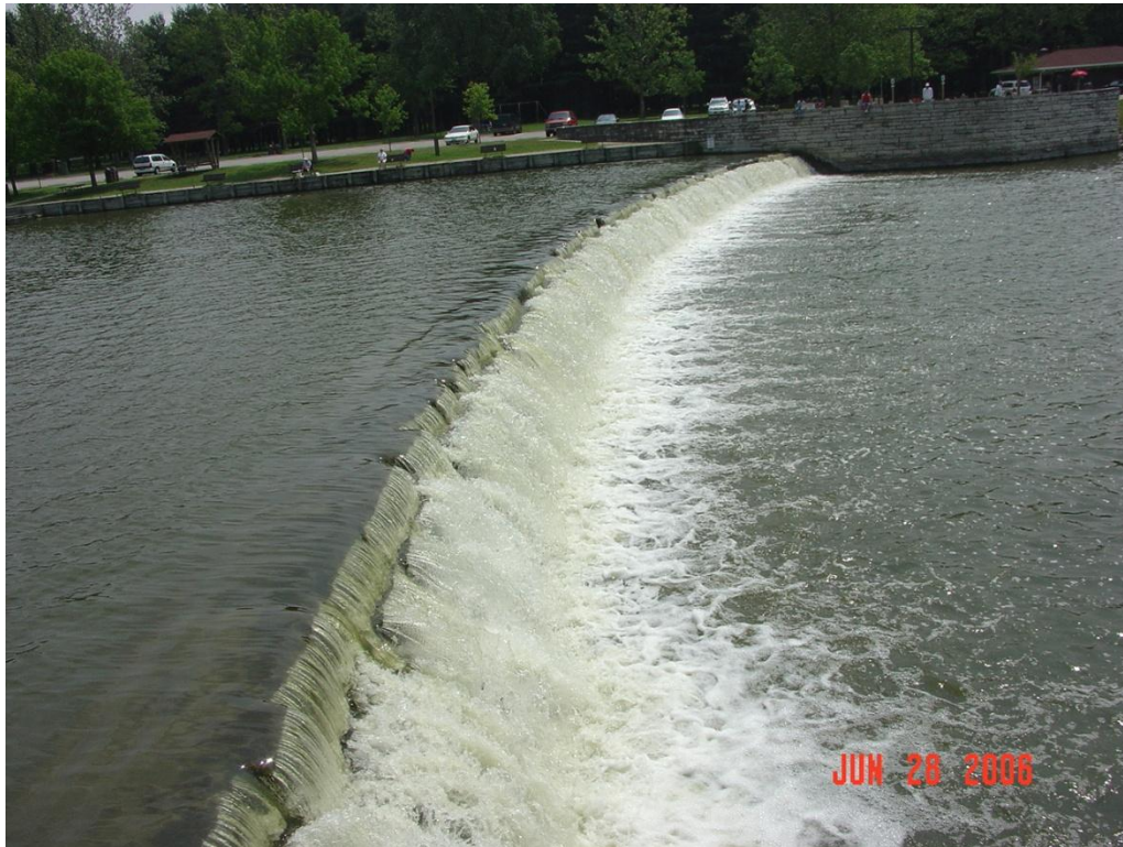
Figure 4: Stratton Dam Spillway
