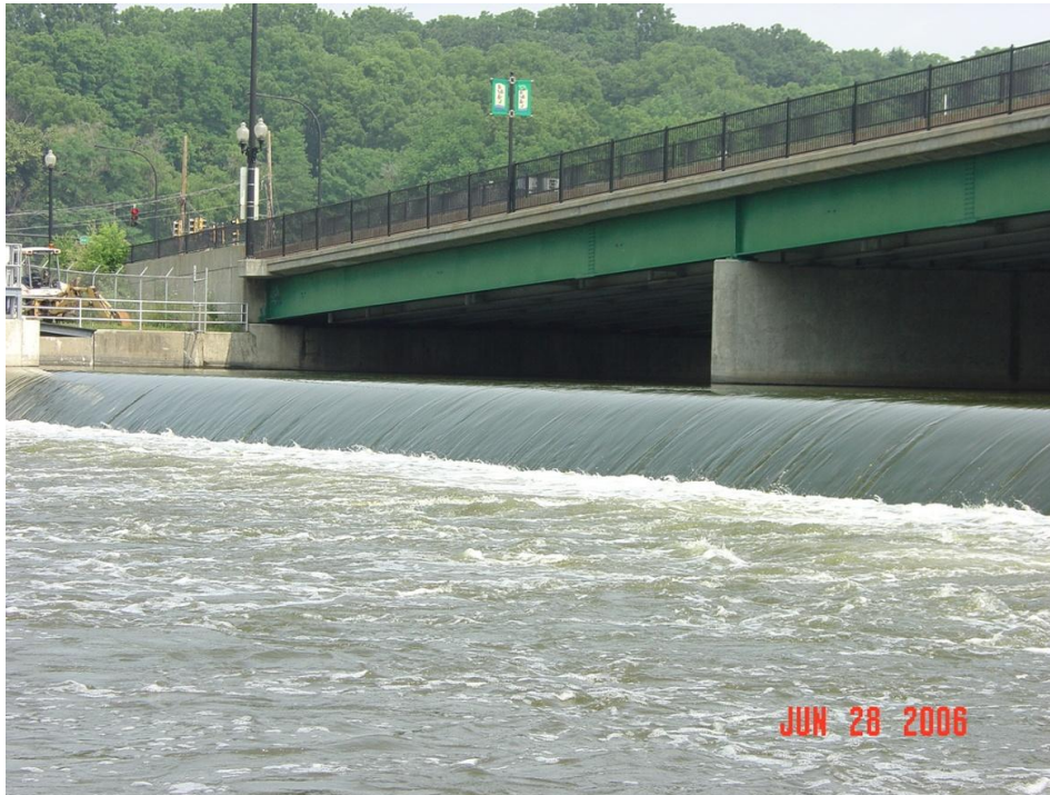
Figure 13: Algonquin Dam Spillway
