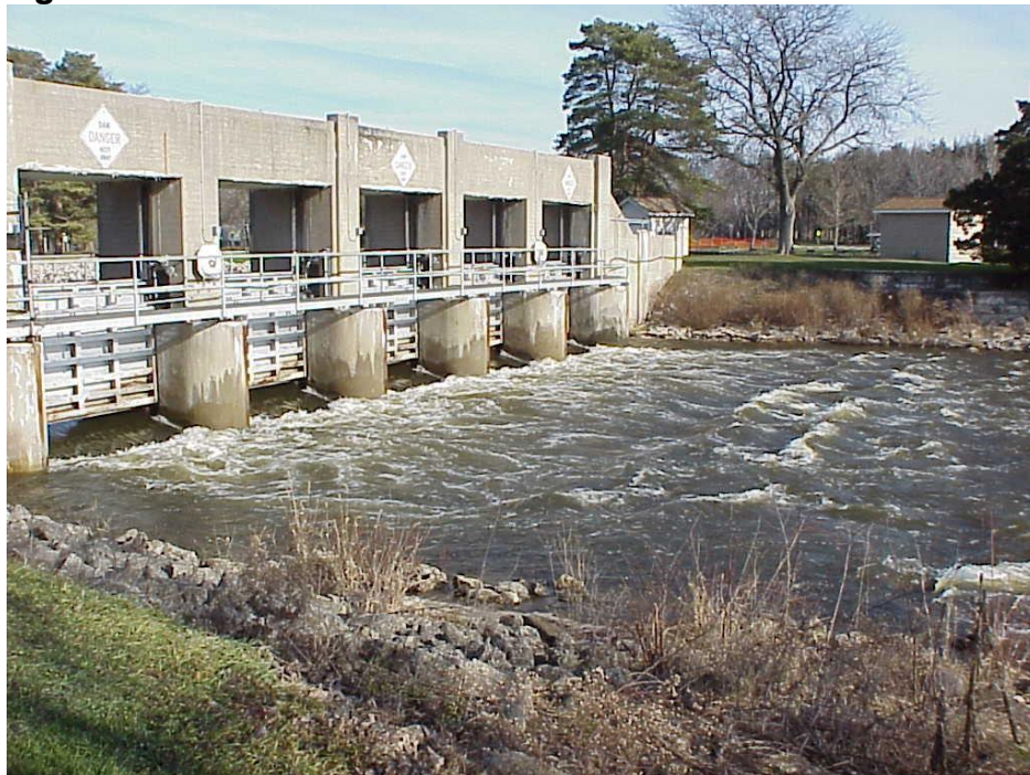
Figure 6: Downstream Side of Stratton Dam Sluice Gates
