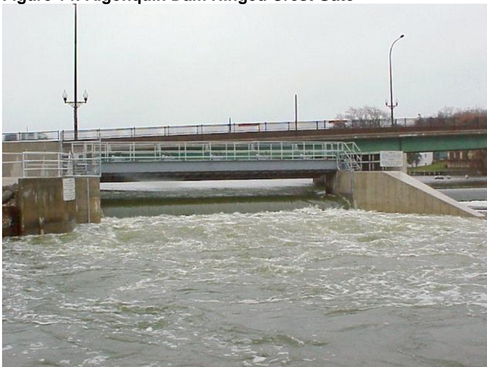
Figure 14: Algonquin Dam Hinged Crest Gate
