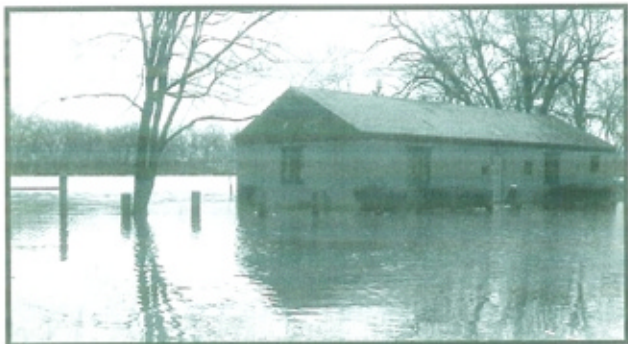
Fox River residential flooding. April 23, 1993.
