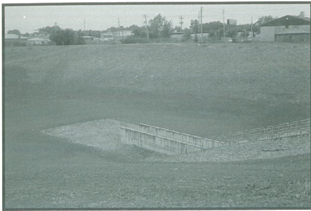
Structure 106. Jack B. Williams Reservoir. Silver Creek. Franklin Park. August 5, 1989.
