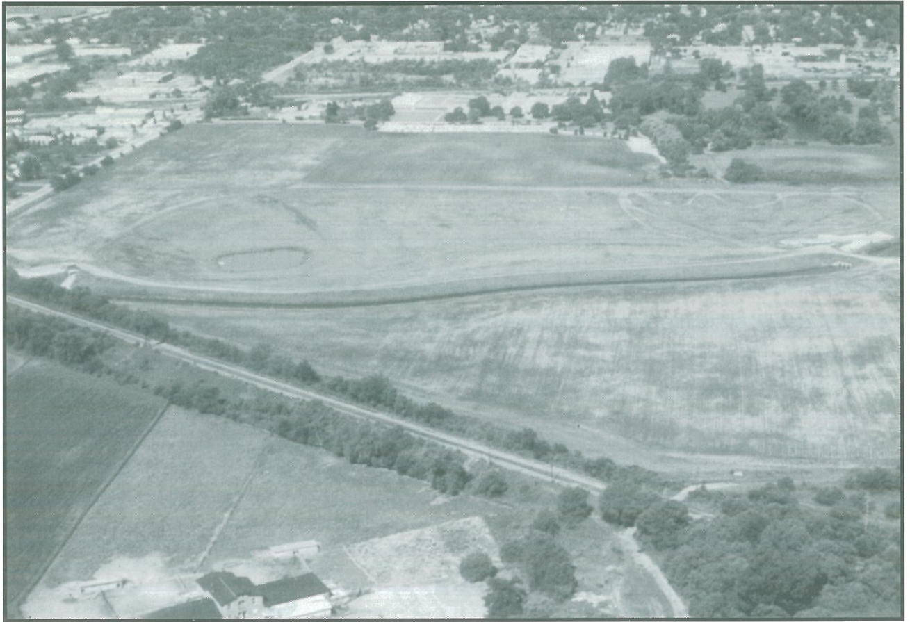
Glenview Reservoir; Structure 32-C. July 1981
