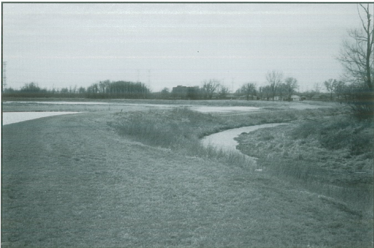
Salt Creek Channel Improvement.
