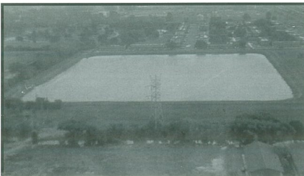
Structure 86. Northlake Reservoir.
