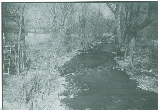
Gaging station on Poplar Creek at Elgin. Villa Street. April 1986.
