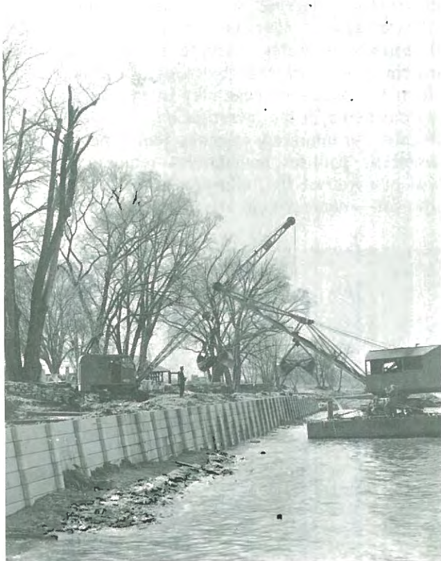
Starved Rock Seawall under construction.
