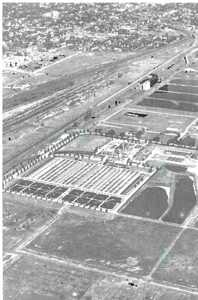
Calumet Treatment Plant.
