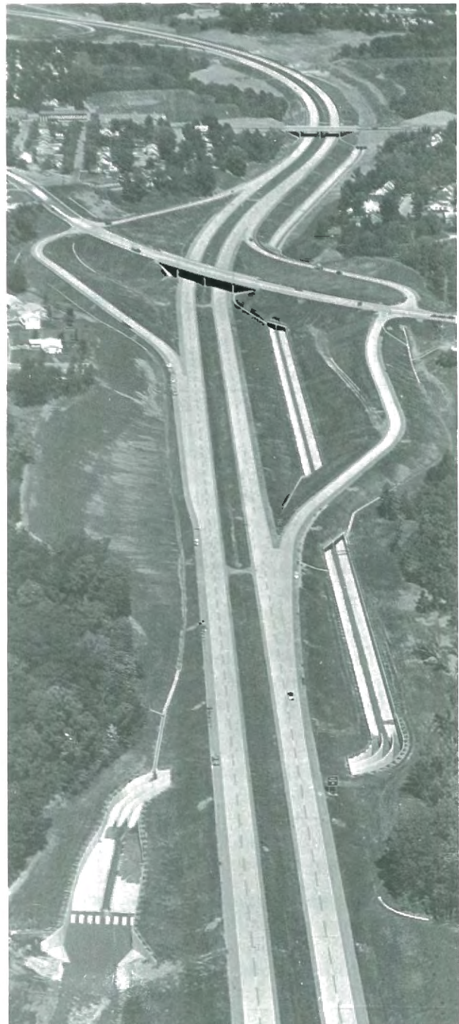
Diversion channel on the West Branch of Dry Run Creek in Peoria.
