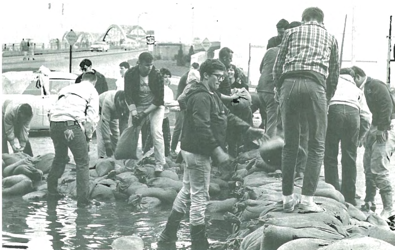
Student volunteers build an emergency sandbag levee during the 1965 Mississippi River flood.
