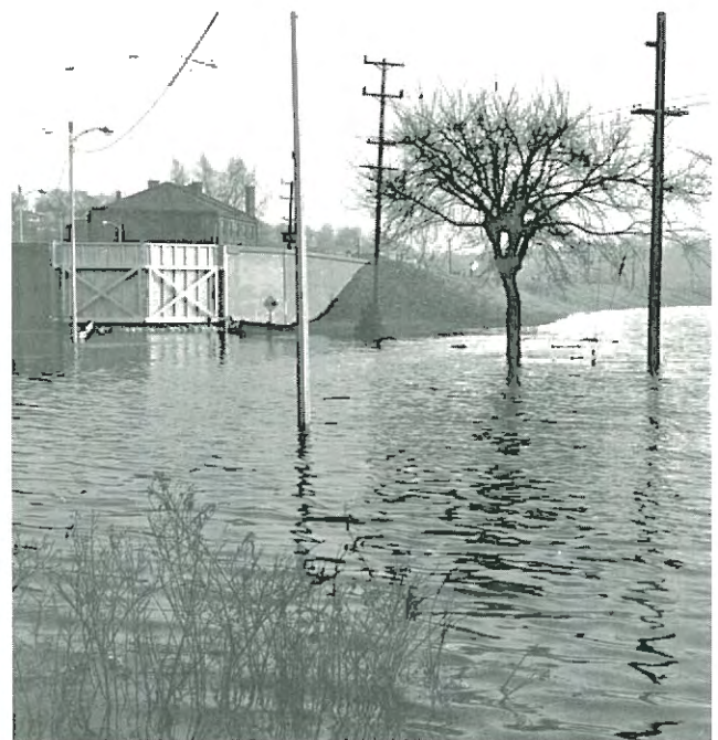
Flood gate protects Galena during the 1965 Mississippi River flood.
