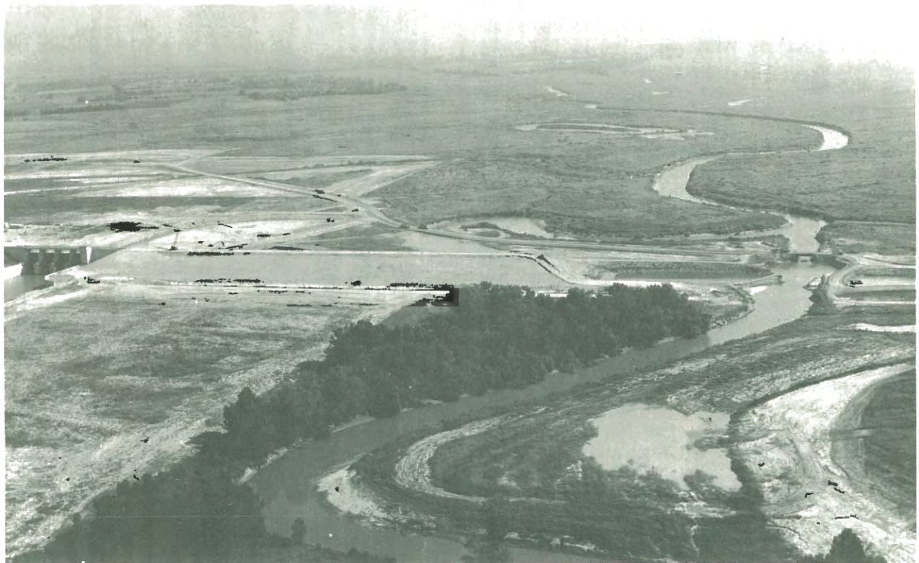
Carlyle Reservoir, Kaskaskia River
