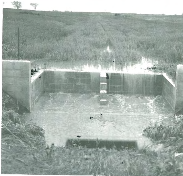
Grass waterway, Fayette County
