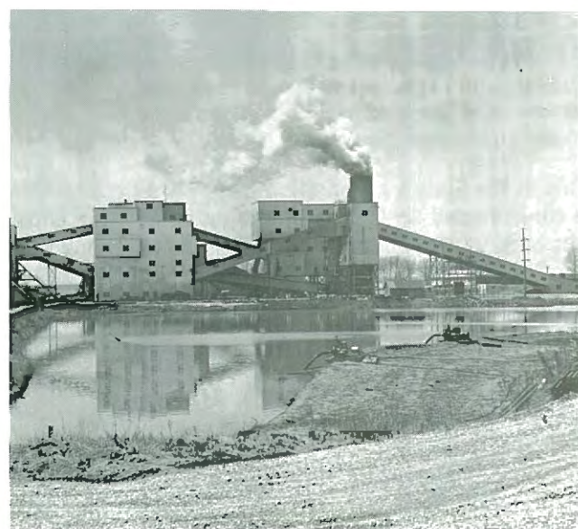
Coal preparation plant.
