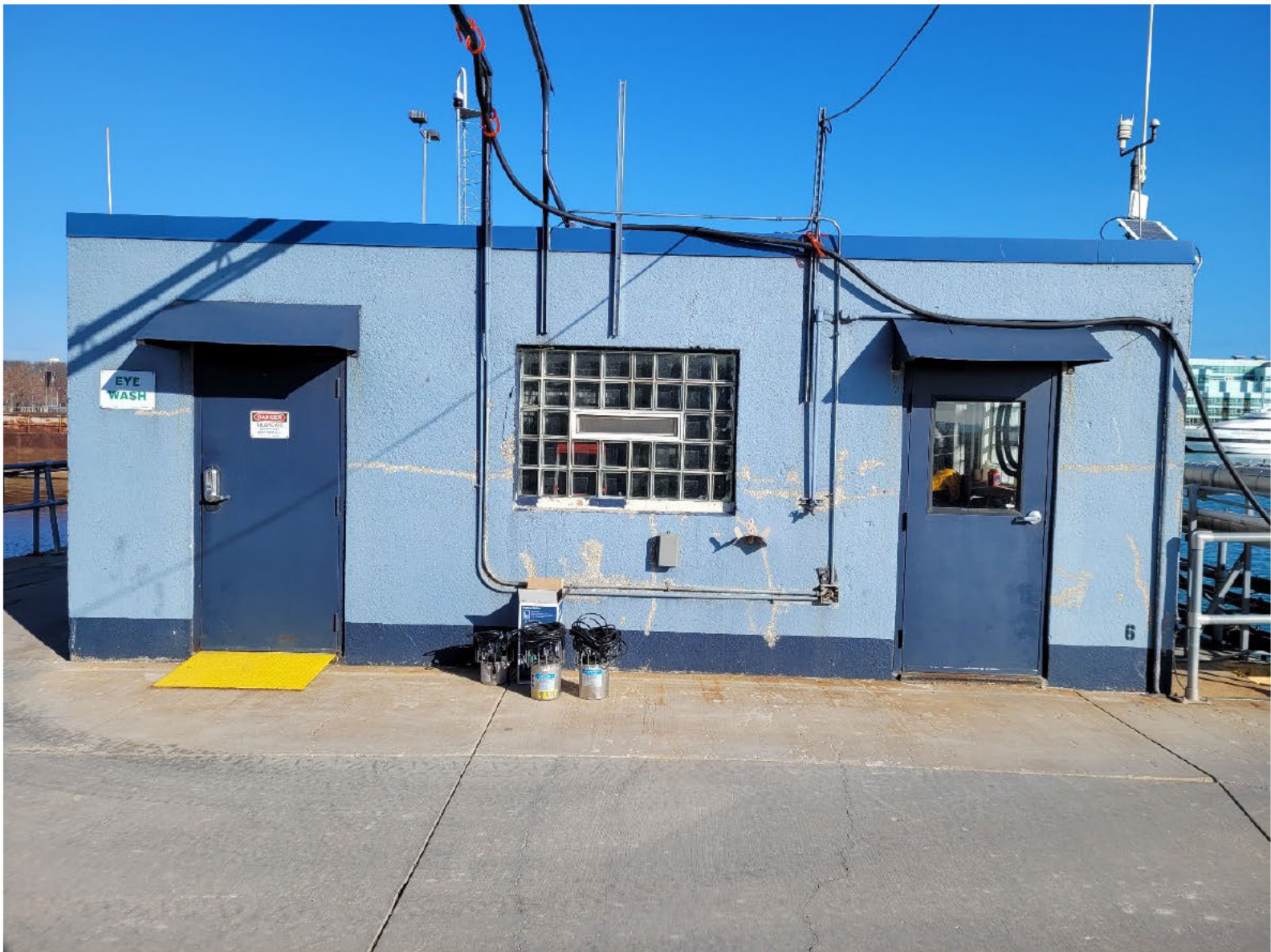
Photo 5. View of the maintenance / tool shop at the western end of the lock chamber at Chicago Harbor, facing north.
