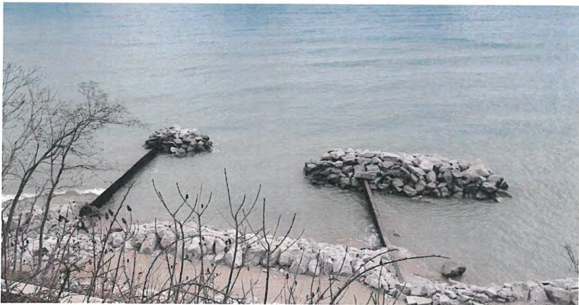
2022 SA Photo – Shows existing condition with lack of sand in the bay
