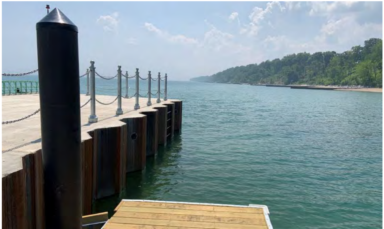
Photo 1: Boat launch area in July 2023 facing southwest
