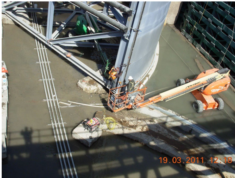
Figure 2: Dewatered gate block with temporary bulk heads in place at Chicago Harbor Lock.
