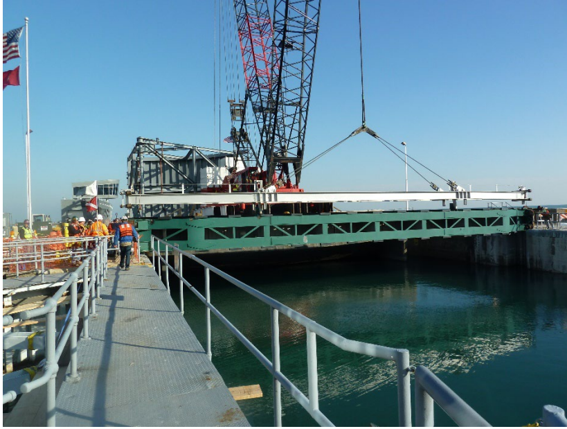
Figure 3: Temporary bulk head placement at Chicago Harbor Lock.
