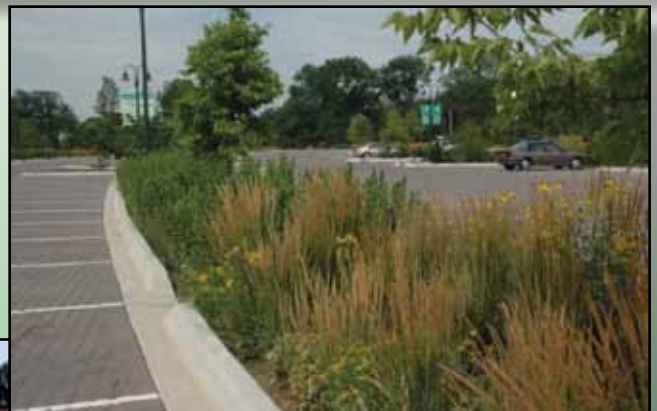
Morton Arboretum parking lot in use... notice holes in pavement to allow rainwater and snow to filter into the gravel base instead of running off into the lake and river.
