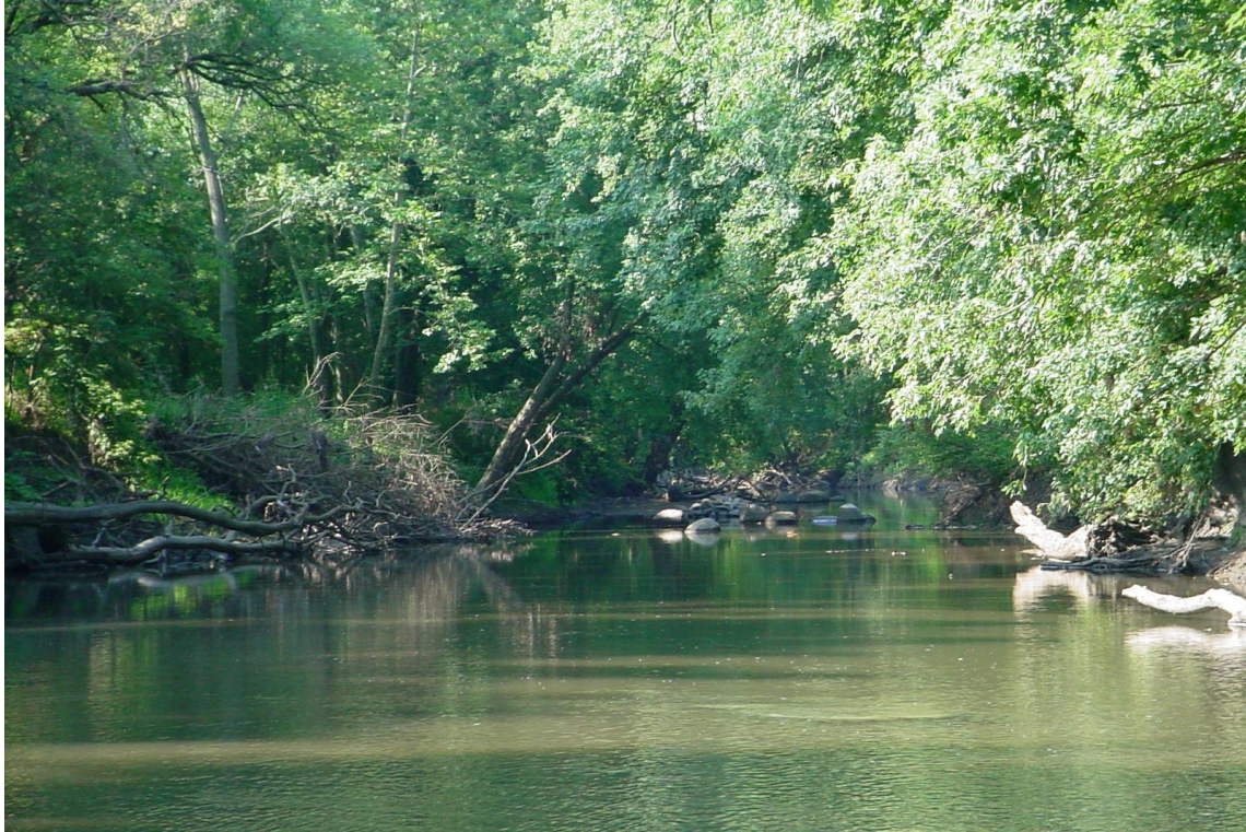
Figure 1. Woody structure (left) and boulder clusters (center) nine months after placement.
