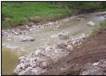
Riffle 5 on Upper North Creek
