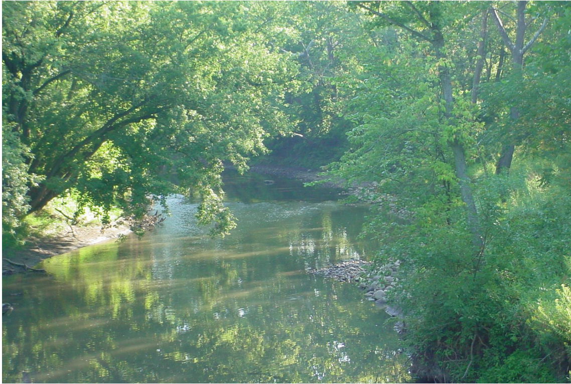
Figure 2. Longitudinal peaked stone toe protection (right), riffle and submerged stone key (center) in Sugar Creek nine months after placement.
