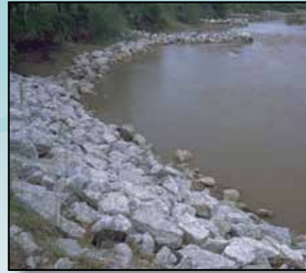
Rock was placed along streams in the Spoon River Watershed to stabilize the banks from eroding.
