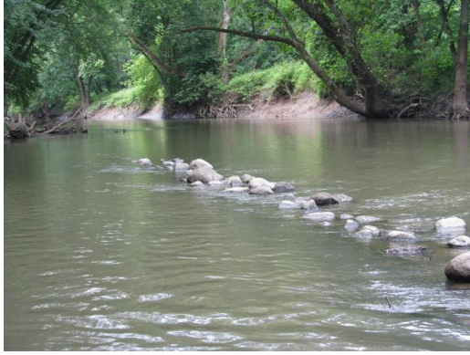
Figure 3. Instream Restoration Longitudinal Stone Habitat Structure.
