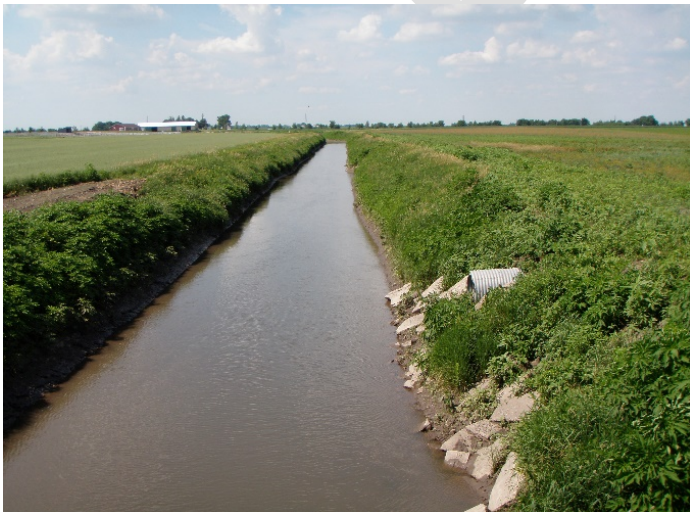
Figure 6. Channelization of an Illinois stream. Photo by S.A. Douglass.
