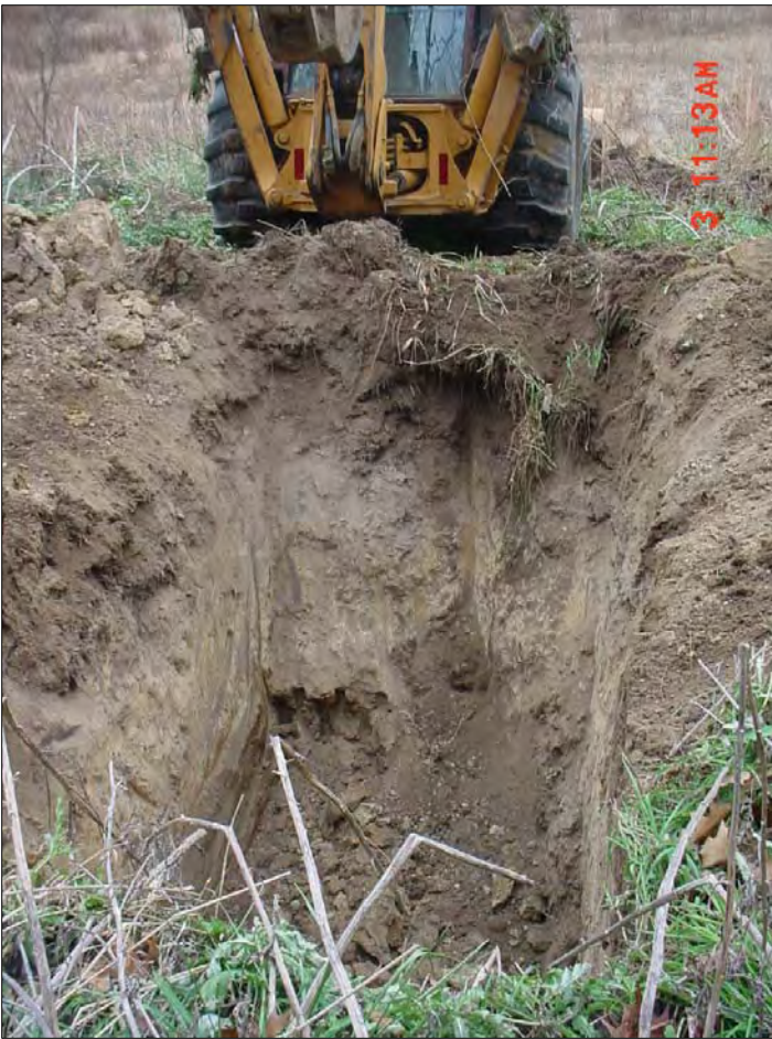
Construction of the reptile hibernacula.
