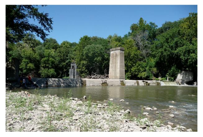
Figure 3. Example of a lowhead dam (<4 m height). Pictured is a lowhead dam on the Vermilion River, Vermilion County, Illinois.
