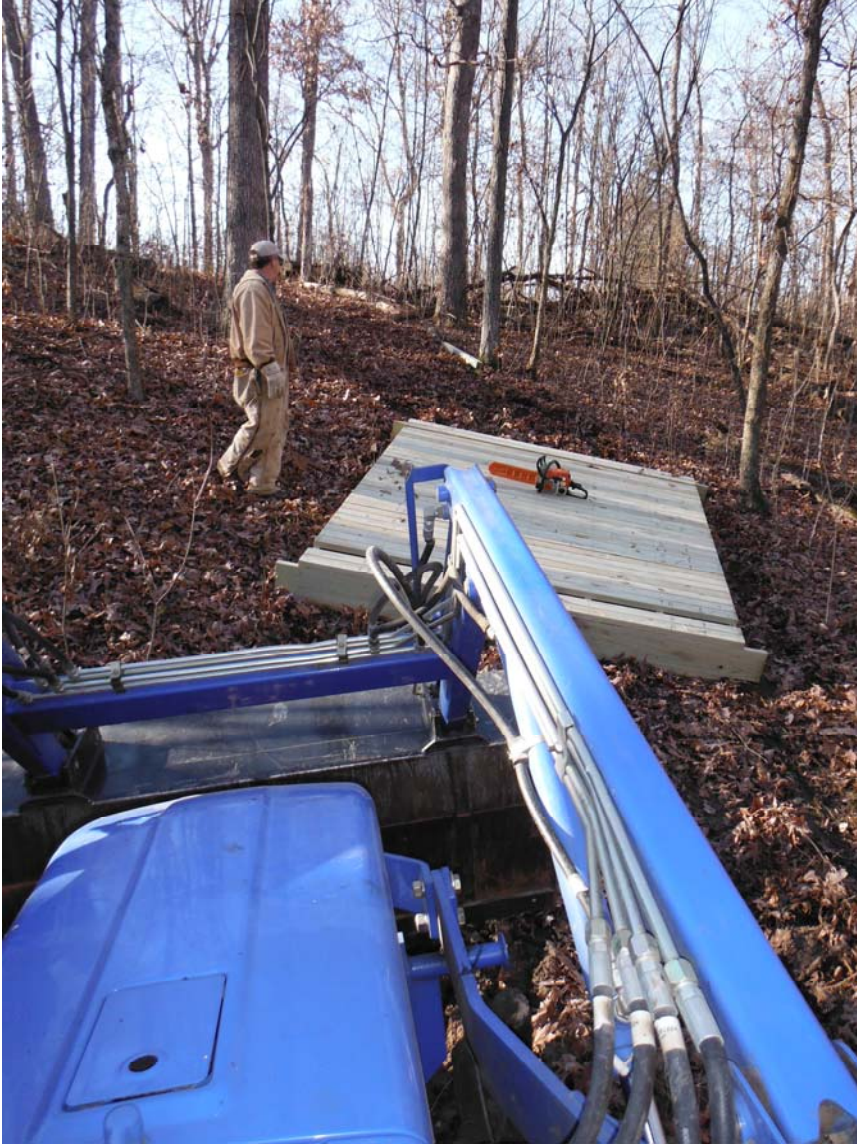
Dragging bridge along trail for placement at waterway
