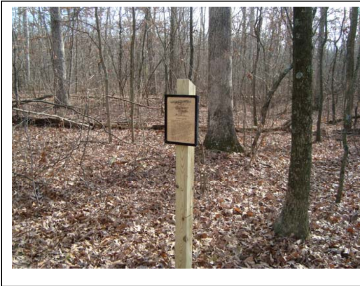
Interpretive signs were positioned on sturdy posts, inserted into 30 inch deep holes in the ground, and installed so that the sign would be at eye-level for an average height adult. Placement of the sign also reflected observable habitat elements.
