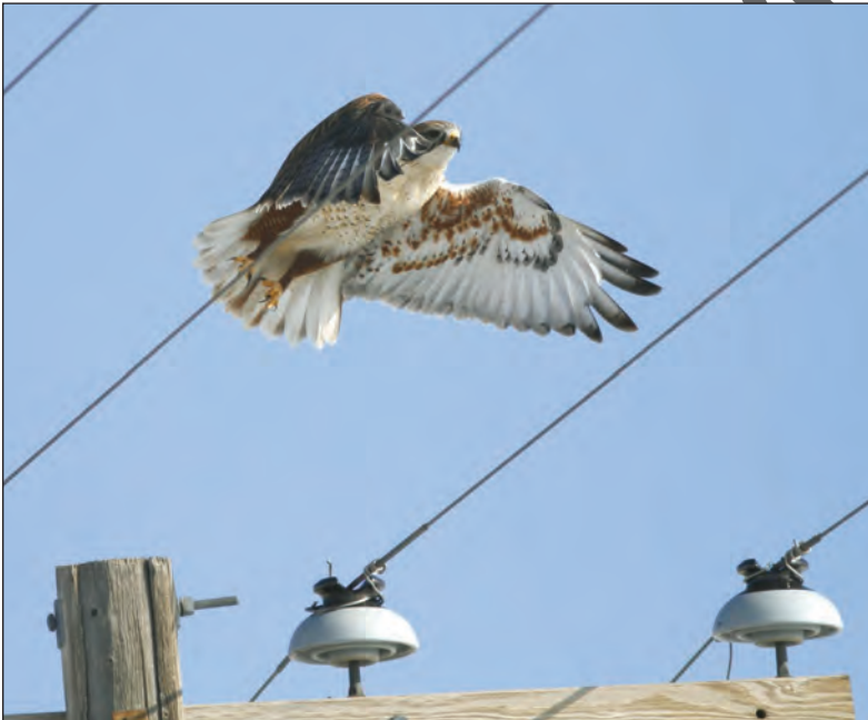
FIGURE 7.1: Utility employee training should include the reasons and methods for reporting bird mortalities, nest management protocols, proper disposal of carcasses, applicable regulations, and the consequences of non-compliance.
