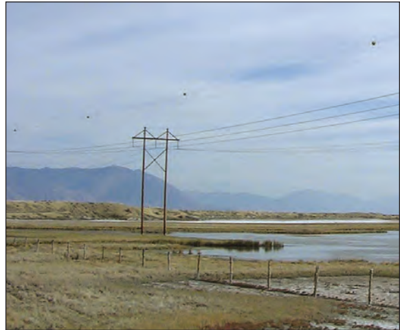
FIGURE 6.9: Aerial marker spheres in use on a power line above a wetland habitat.
