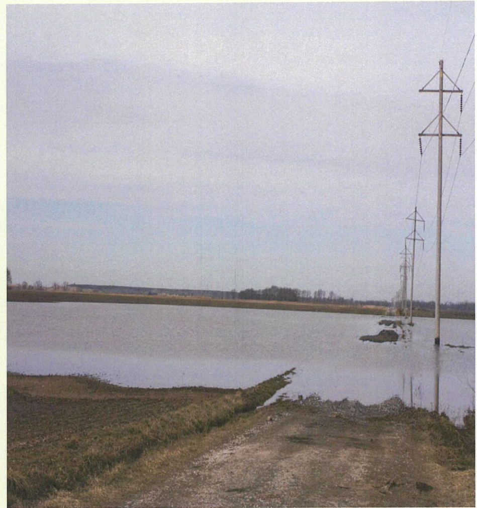
Same field after subsidence
