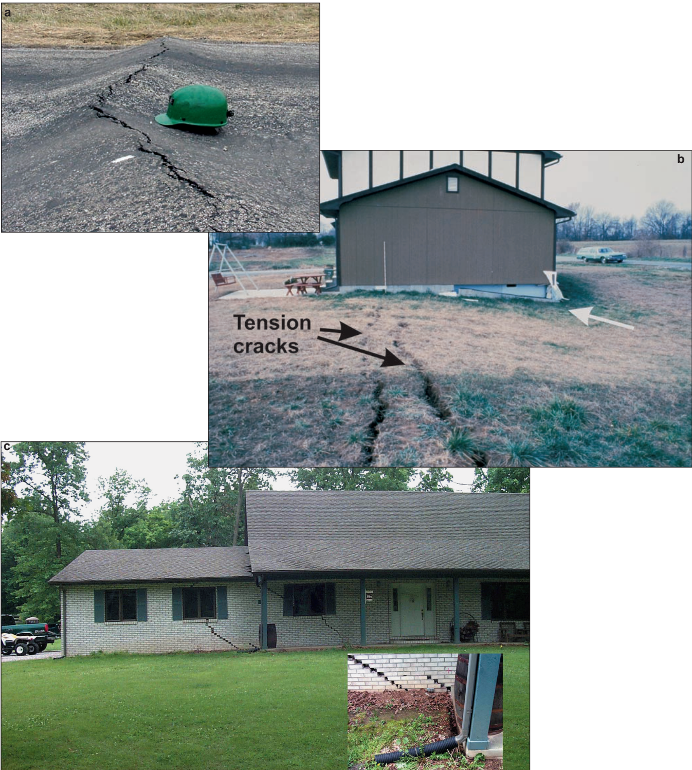
Figure 14 Photographs illustrating the sag subsidence event and features shown in figure 13. (a) Compression ridges formed in the road (feature R) as the result of ground movement (compression) associated with coal mine subsidence. (b) Tension cracks form in the ground surface extending through a home (feature H1); the foundation has settled at the house corner close to the center of the sag. (c) The brick-sided house (feature H2) in the tension zone shows downward bending (compare roof lines). The left side of the home is closest to the sag center and has dropped down. Inset: Ground has pulled away from the porch toward the sag center (left).
