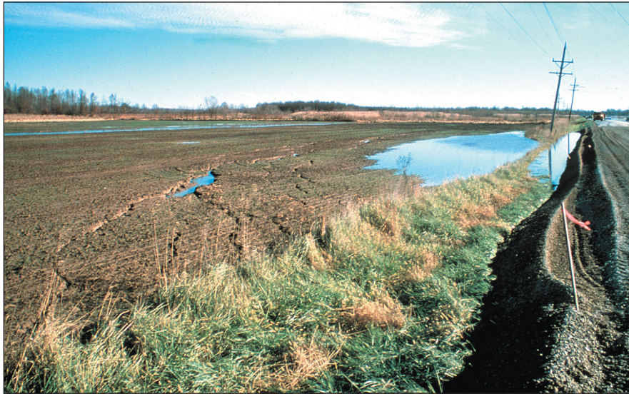
Figure 18 Ponding created by sag subsidence. Note the tension cracks around the edge of the depression.
