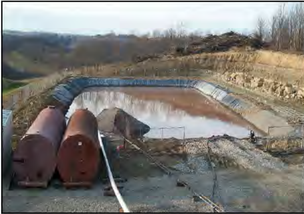
An on-site lagoon is one option for temporary storage of drill cuttings/fluids and flowback water.
