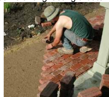
Dedicated Save the Prairie Volunteer building the walkway with your bricks
