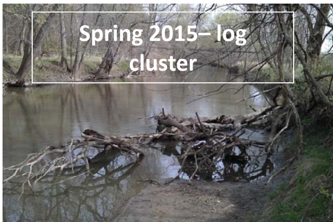
Figure 11. A Log Cluster, which provides a diverse complex of habitat. The woody debris is cabled to a tree along the streambank to secure it in place. Photos courtesy of Illinois Natural History Survey staff.
