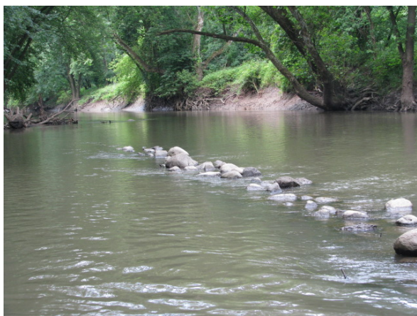
Figure 3. Instream Restoration Longitudinal Stone Habitat Structure (photo credit: IDNR's Contaminant Assessment Section).
