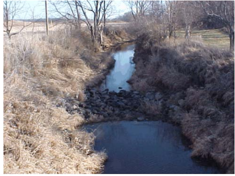
Figure 2. First rock riffle grade control structure downstream of the 1100 N bridge.
