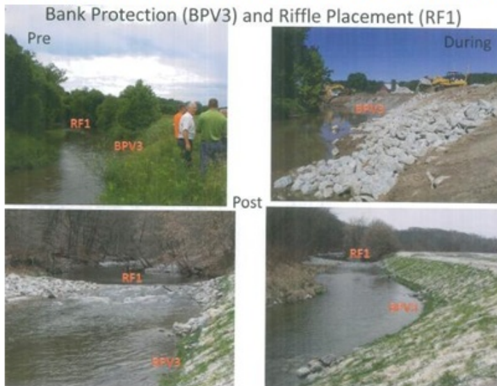
Example of the Kickapoo Creek Riffle/Bank Protection
