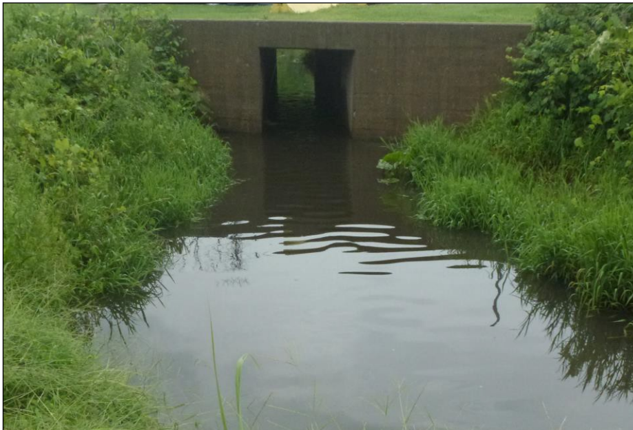
EXHIBIT 7 DEAD CREEK CS- F ( LOOKING EAST; 7 AUGUST 2018 )
