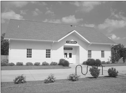
TUNNEL HILL STATE TRAIL SITE OFFICE
