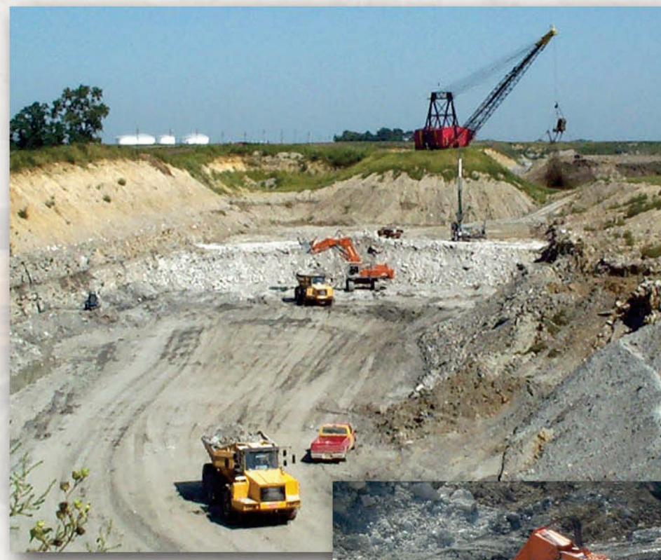
Loading and Hauling Blasted Rock
