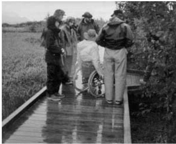
Figure 25--This boardwalk relies on pilings for support. Helical earth anchors can also support the structure.
