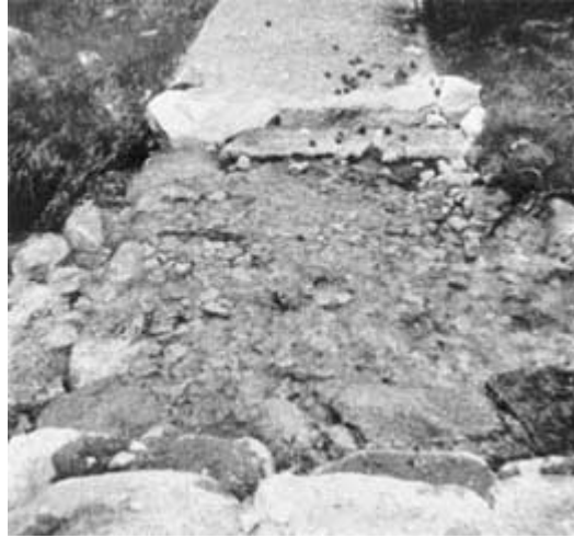
Figure 28--Wide cross drain and causeway
