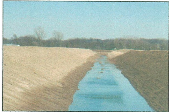
Levee rehabilitation work near Caseyville, Illinois.
