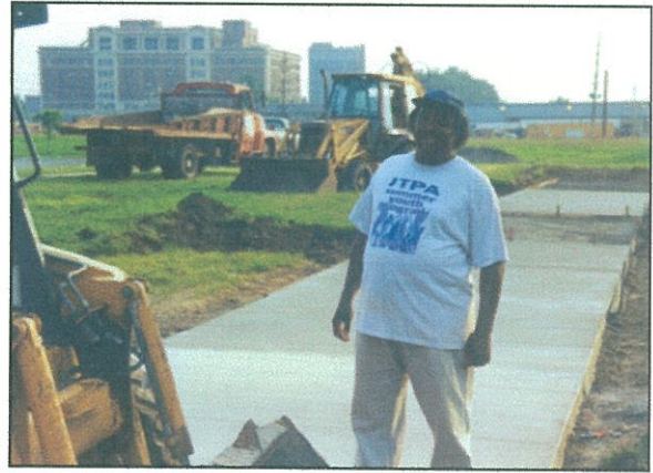
Trail construction in East St. Louis, Illinois
