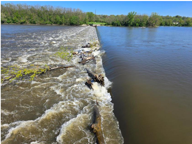
Figure 8 - Steel Dam Looking North from Southern Bank at Park (Prairie 2024).
