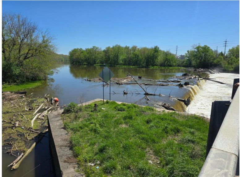
Figure 7 - Sears Dam Looking Upstream from Highway 67 Bridge (Prairie 2024).
