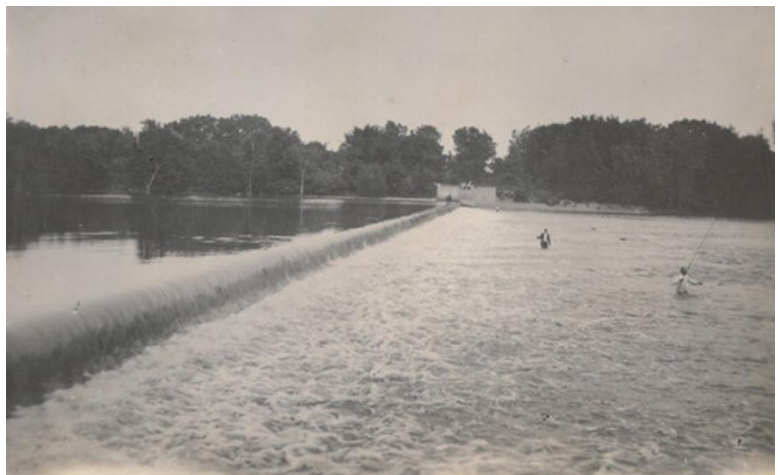
Figure 6 - Looking south along the Steel Dam from Vandruff Island, July 26, 1904
