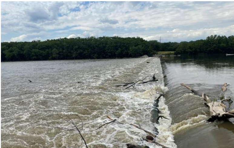
Figure 20. Steel Dam, looking from river left across towards Vandruff Island. June 13, 2024. Location: 41.459772, -90.547531
