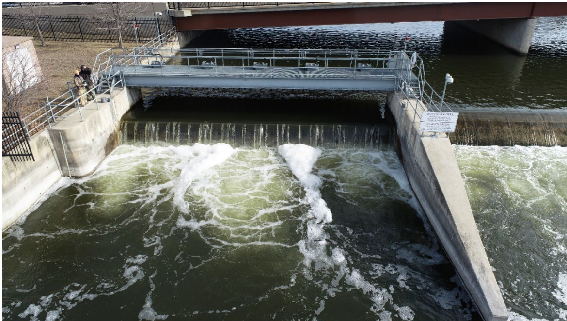
Figure 13: Algonquin Hinge Crest Gate
