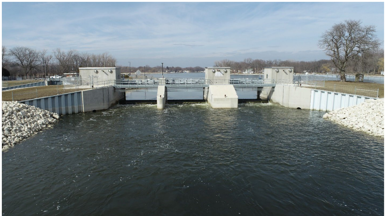
Figure 5: Downstream Side of Stratton Torque Tube Gates
