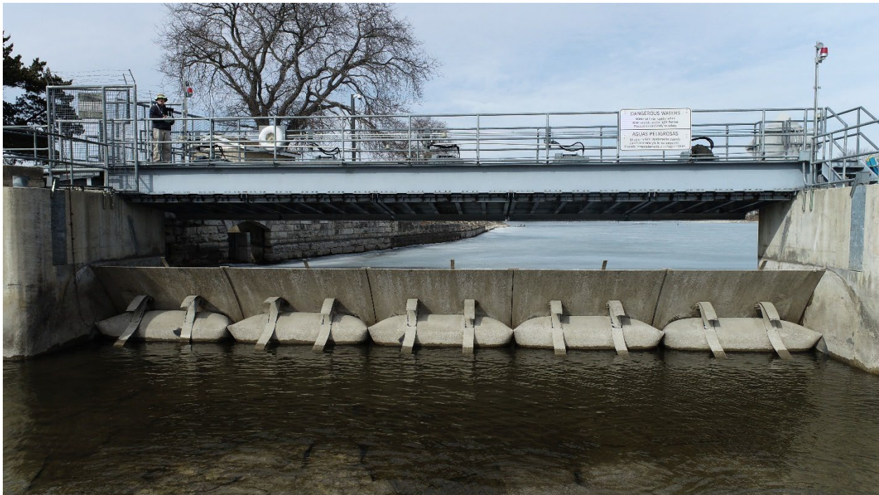
Figure 6: Stratton Dam Hinged Crest Gate
