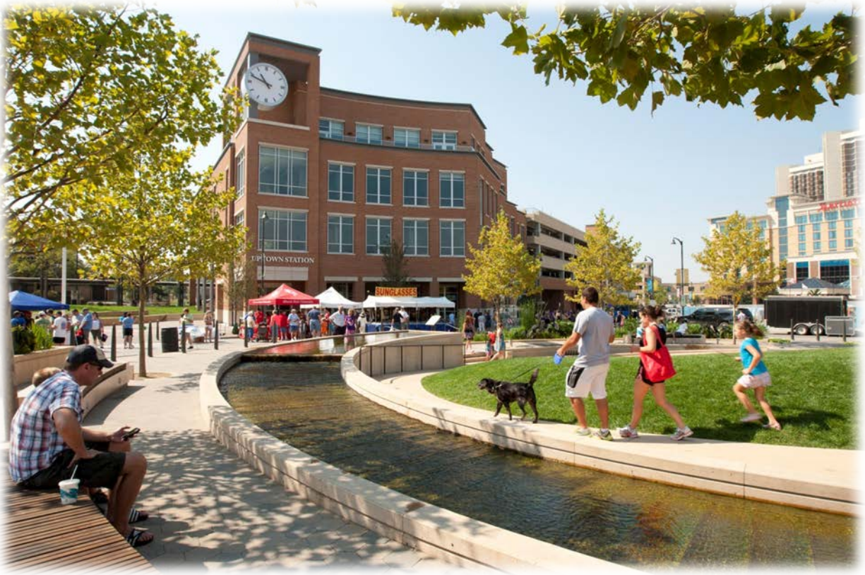
The Normal, IL roundabout project combines green and gray infrastructure to provide an appealing community focal point with stormwater management. Photo credit: Scott Shigley
