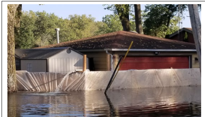
Figure 2.16 Home in McHenry County using sandbags, a floodwall and pumps to protect from shallow flooding.
