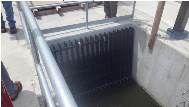
All new lock and intake structure sluice gates have been installed and are fully functional. Lock extension is compete and has been fully functional since May 1, 2015.
