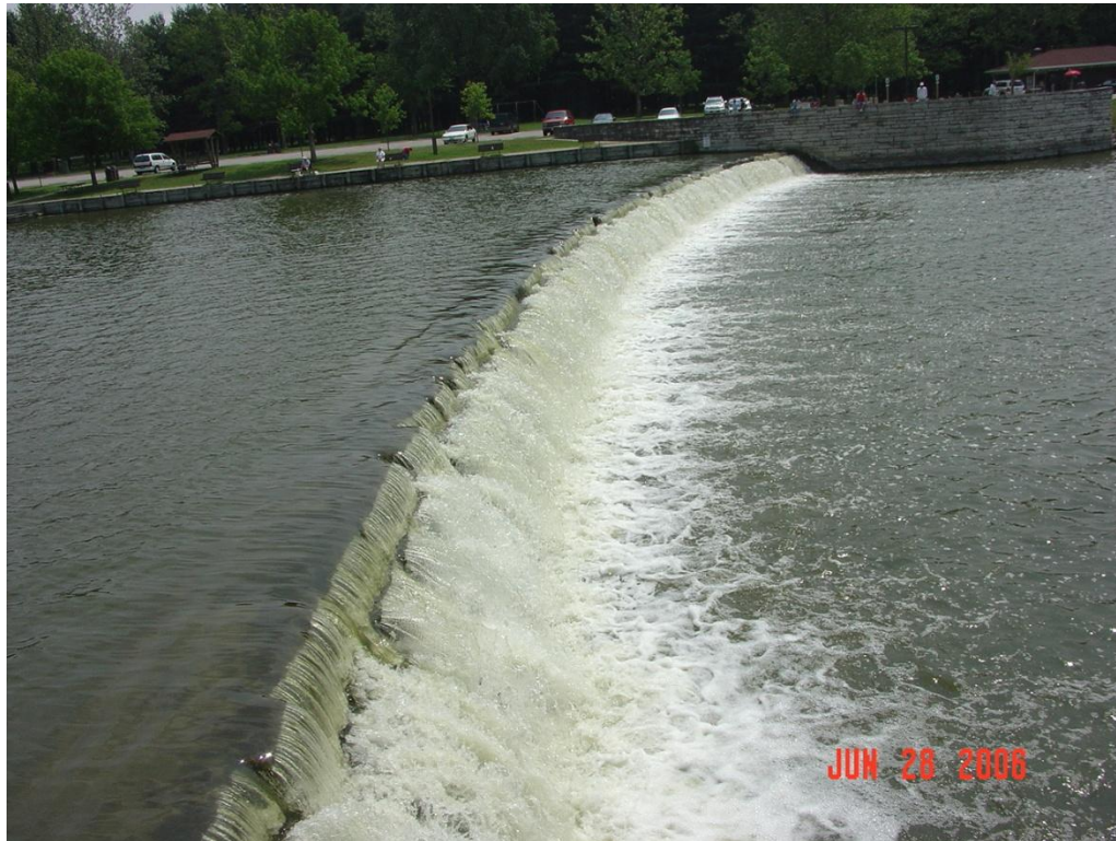
Figure 4: Stratton Dam Spillway
