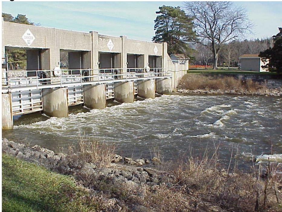
Figure 6: Downstream Side of Stratton Dam Sluice Gates
