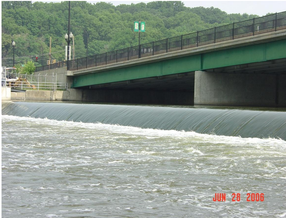
Figure 13: Algonquin Dam Spillway
