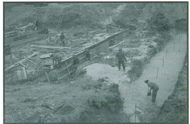
Structure 27, Bannockburn Reservoir: Deerfield.
