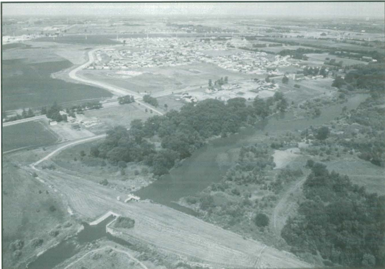
Naperville Reservoir, DuPage River: July 1981
