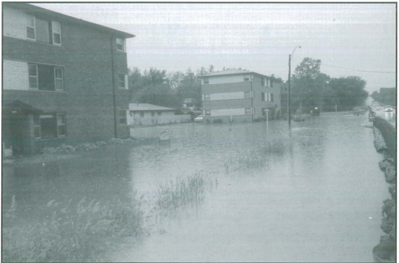
Hickory Hills. Looking west along the south side of 87th Street at 83rd Avenue. June 8, 1993.
