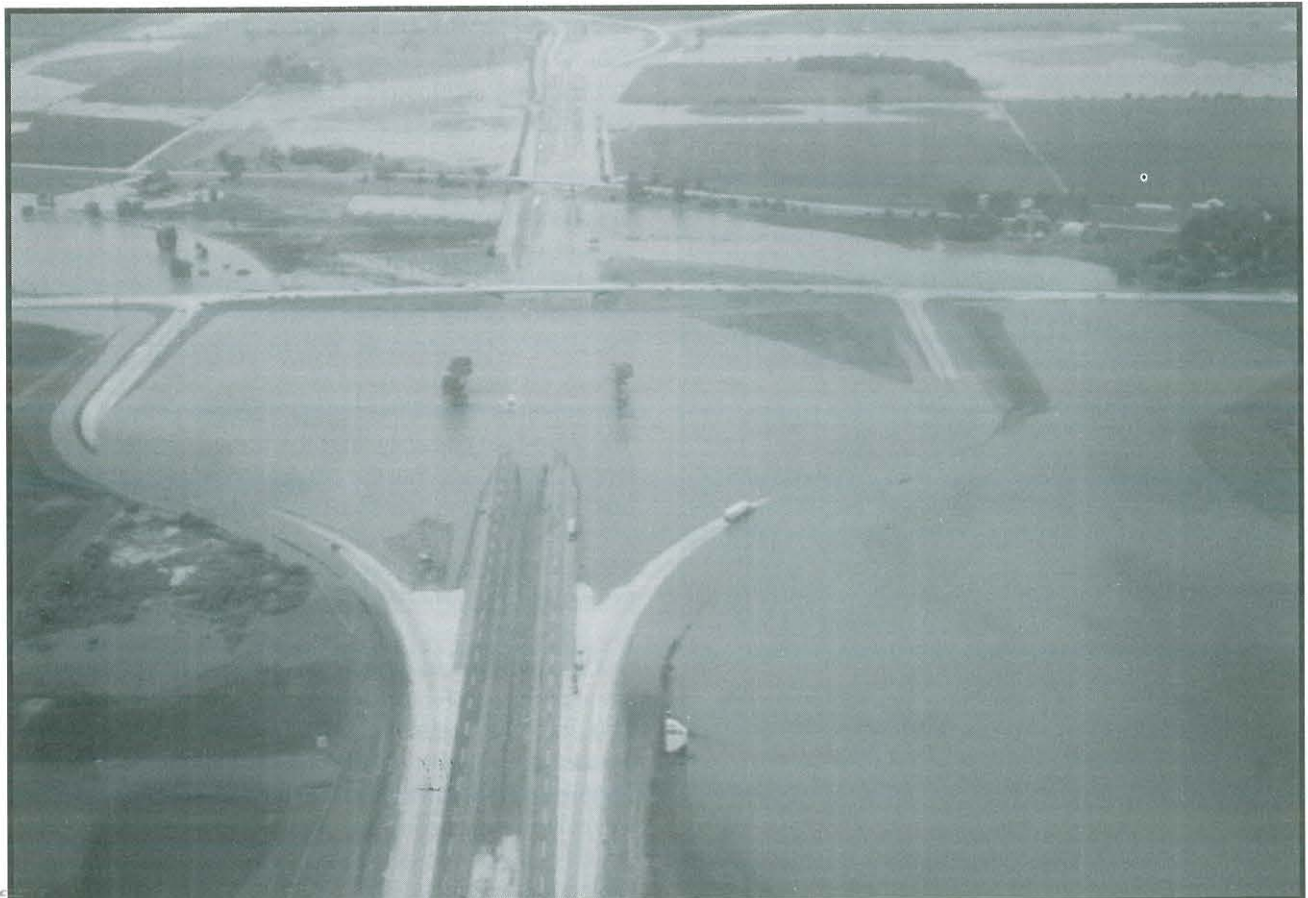
Aerial view of flooding in Kane County, Ill. Looking west at Orchard Road. July 18, 1996. (Photo by Chris Dagiantis, Courtesy of Paul Schuch. Kane County Development Department.)
