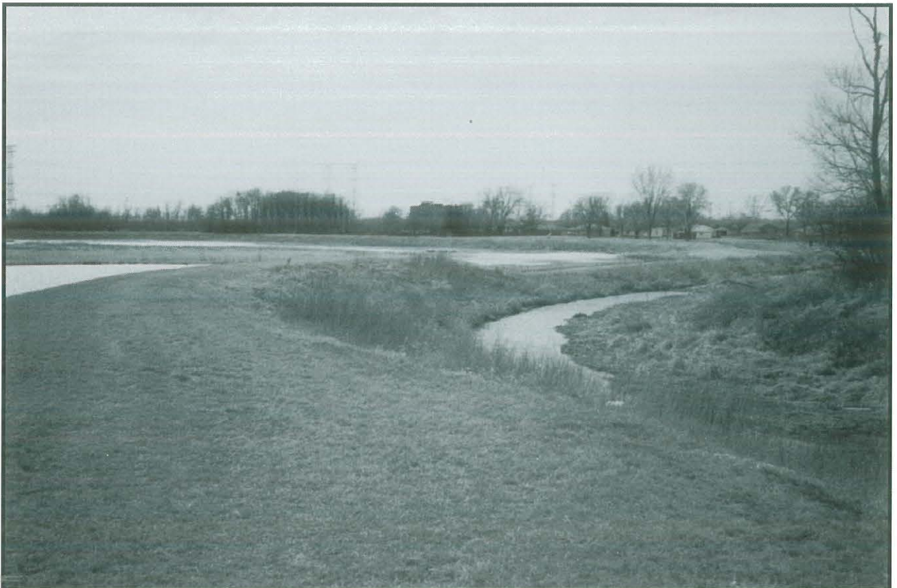
Salt Creek Channel Improvement.
