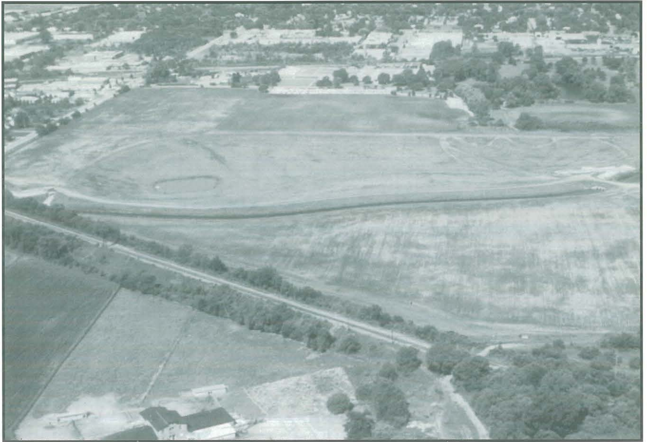
Glenview Reservoir, Structure 32-C. July 1981
