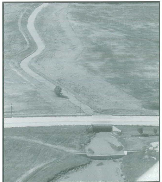
Techy channel improvement. July 1981
