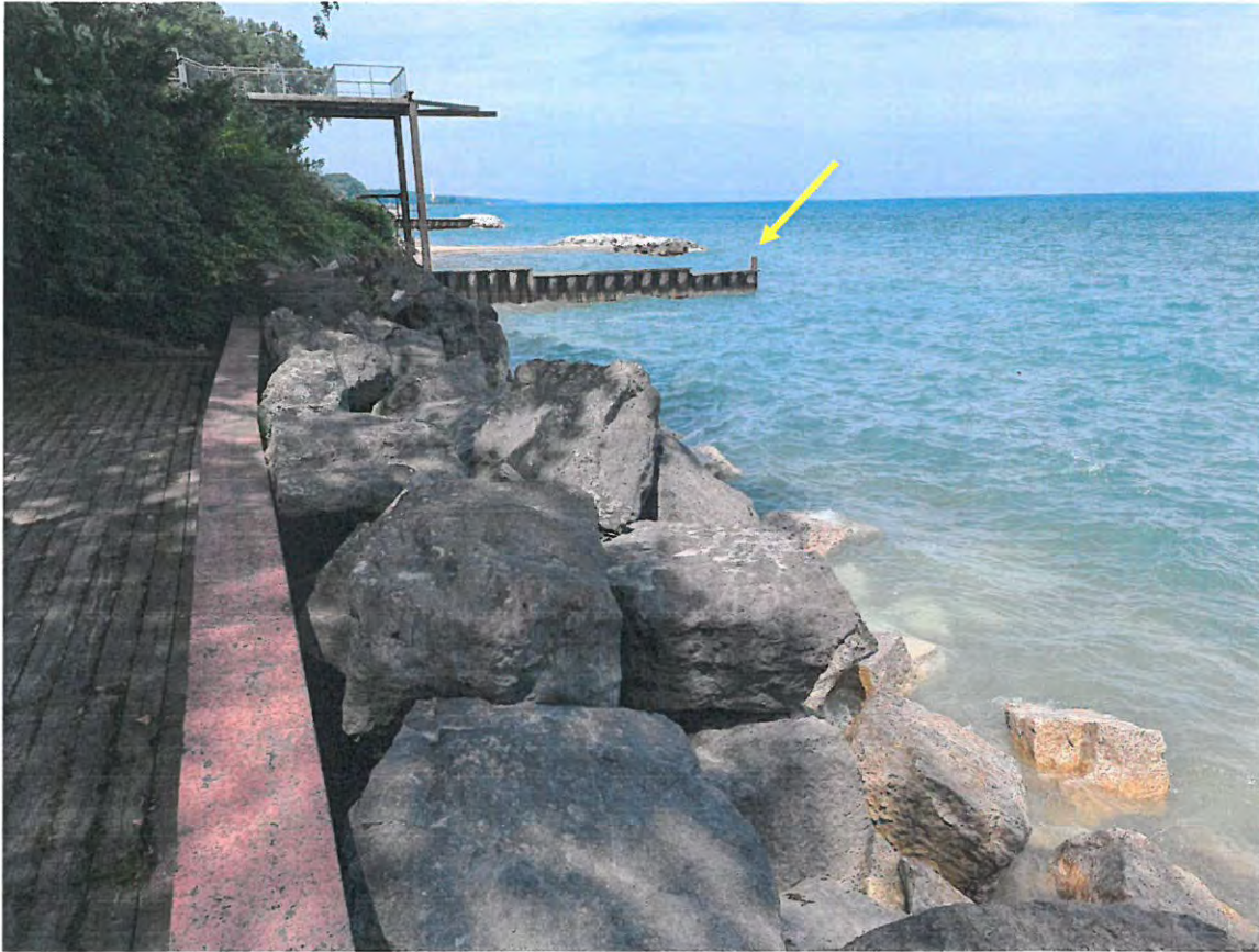
2025 SA Photo looking north along the existing revetment to the adjacent steel groin (yellow arrow)
