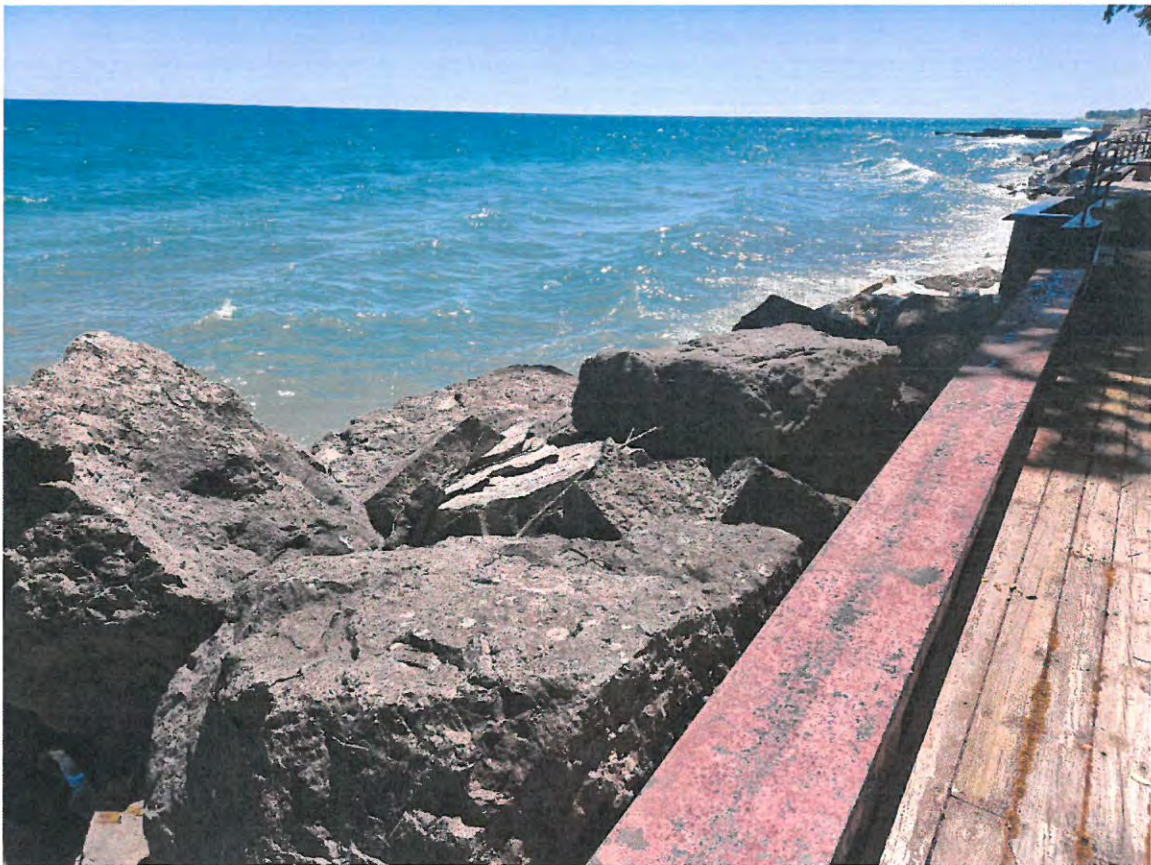
2022 SA Photo looking south shows existing limestone revetment a steel seawall cap
