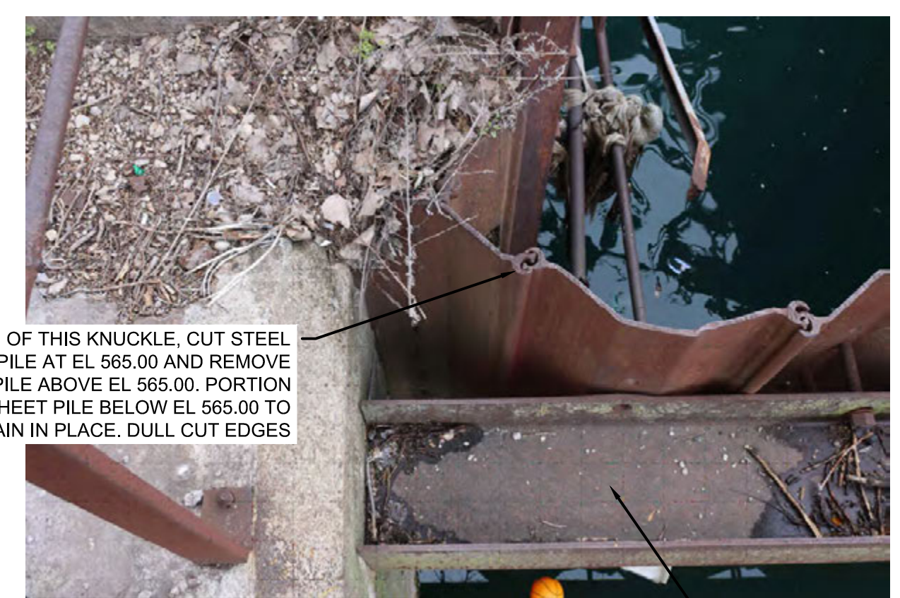
2 PHOTO: NORTH WALL NOT TO SCALE NOTE: 1. PHOTO TAKEN LOOKING EAST.
