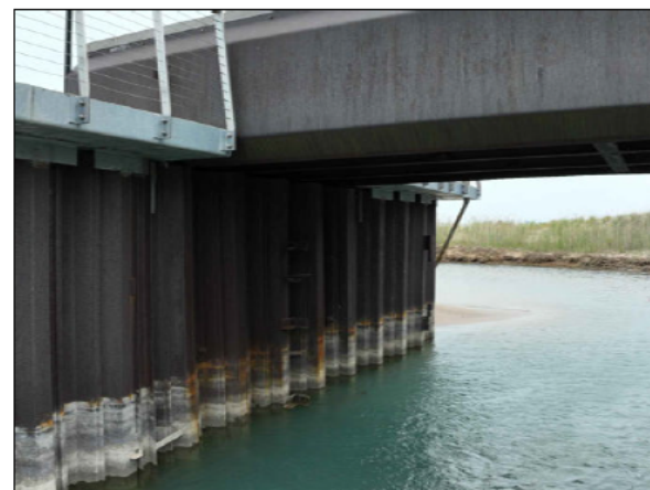
PHOTO: 9 DIRECTION: NORTHWEST DATE TAKEN: 06-16-2023 NOTES: EXISTING BRIDGE
