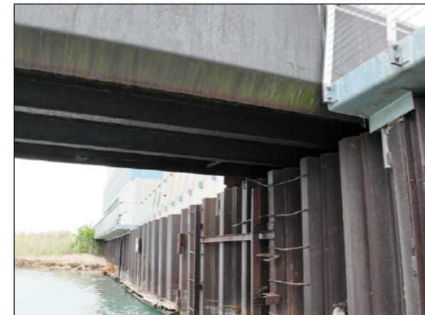
PHOTO: 10 DIRECTION: SOUTH DATE TAKEN: 06-16-2023 NOTES: EXISTING BRIDGE ABUTMENT
