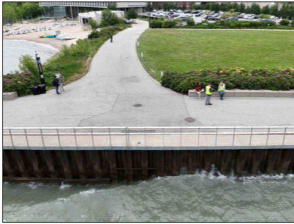
PHOTO: 13 DIRECTION: WEST DATE TAKEN: 06-16-2023 NOTES: SOUTH OUTFALL
