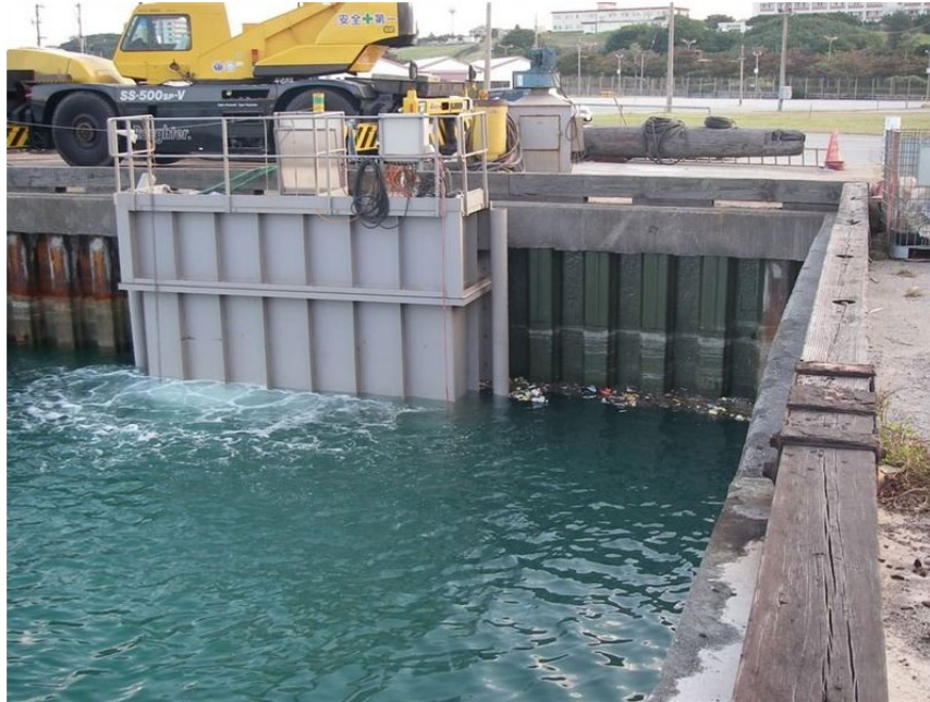
Figure 3.1: Temporary Mobile Sheet Pile Cofferdam System (Acotec)
