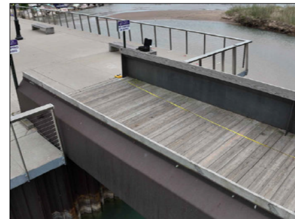
PHOTO: 11 DIRECTION: NORTHWEST DATE TAKEN: 06-16-2023 NOTES: EXISTING BRIDGE DECK
