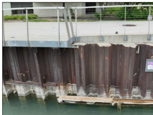
PHOTO: 6 DIRECTION: WEST DATE TAKEN: 06-16-2023 NOTES: EX. SHEET PILE & WALER
