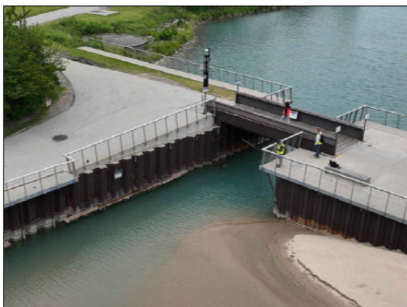
PHOTO: 3 DIRECTION: NORTHWEST DATE TAKEN: 06-16-2023 NOTES: AERIAL OBLIQUE
