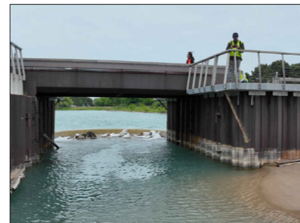
PHOTO: 12 DIRECTION: NORTH DATE TAKEN: 06-16-2023 NOTES: EXISTING BRIDGE
