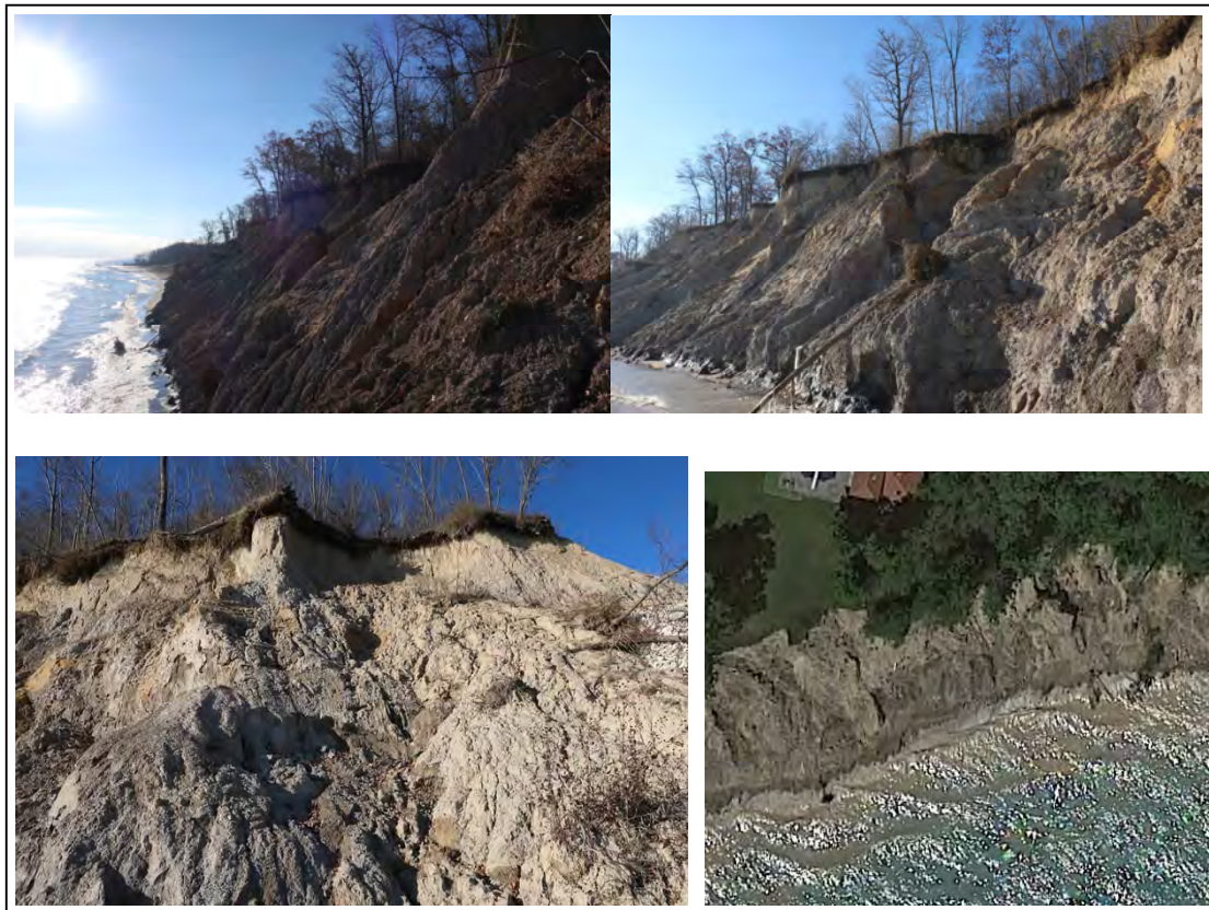
Figure 2 - 663 Circle Lane Existing Slope Photos
