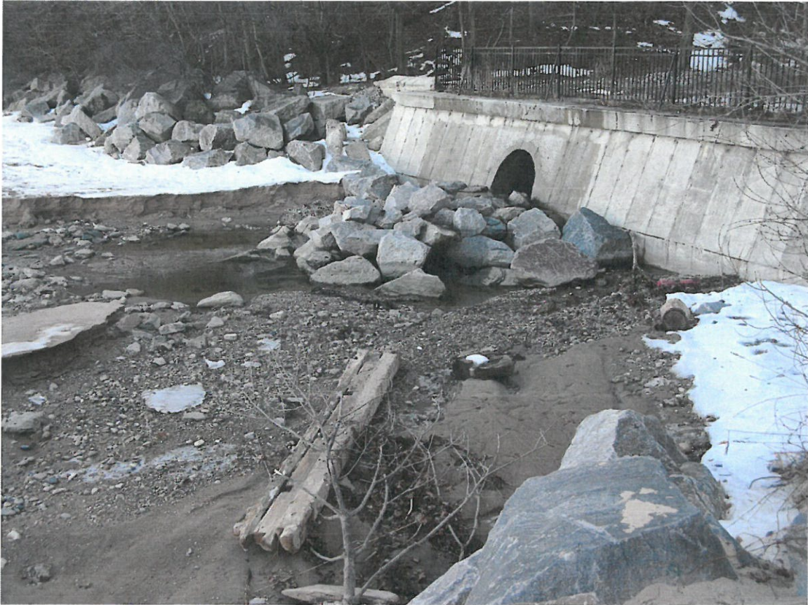
2008 SA Photo showing the Fisher Lane stormwater outfall and washout to the beach
