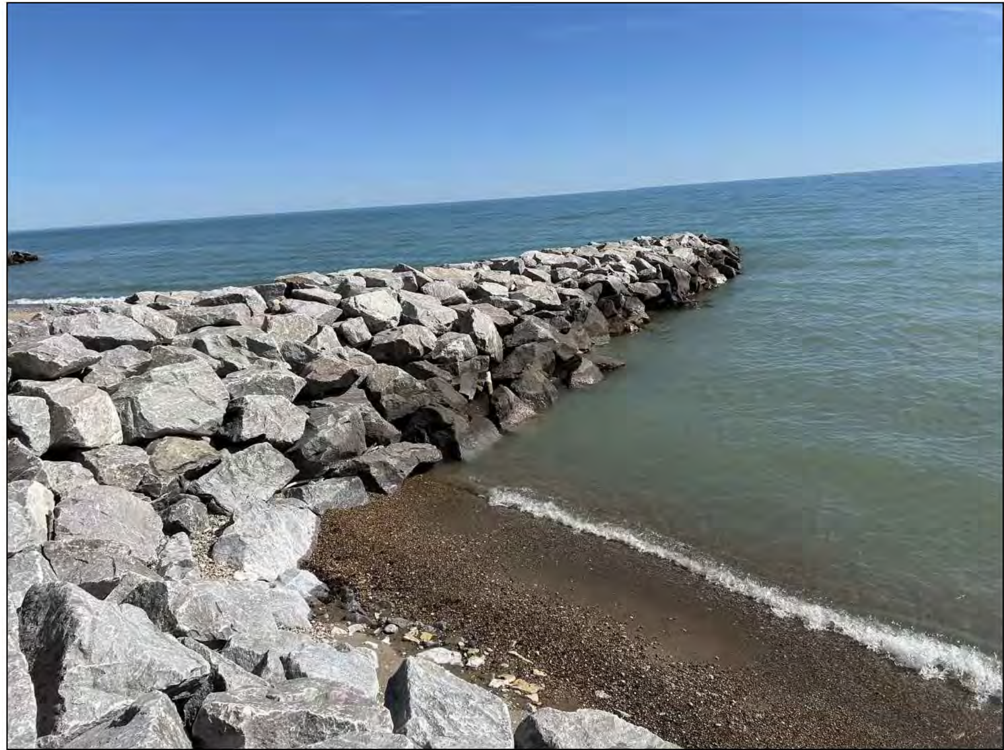
PHOTO 1: LOOKING NORTHEAST AT NEIGHBORING NORTH ARMOR STONE GROIN.
