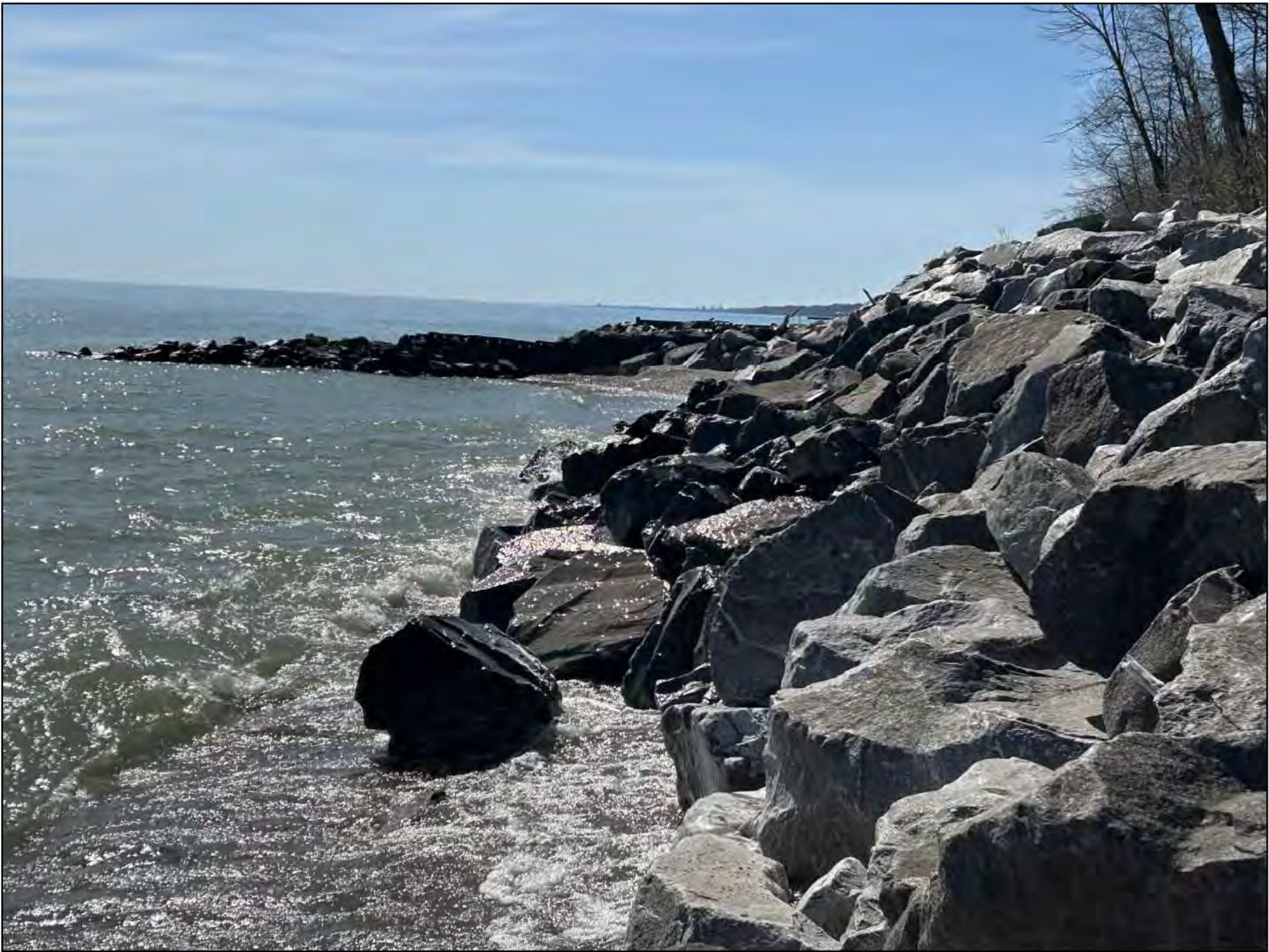
PHOTO 2: LOOKING SOUTHEAST AT DISPLACED REVETMENT ARMOR STONE.
