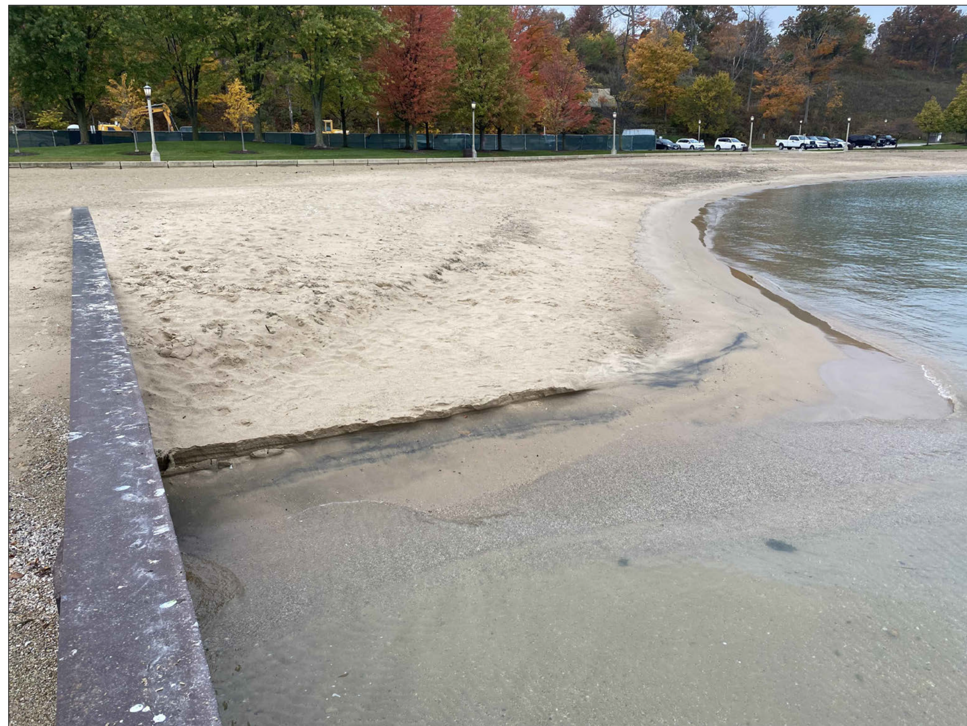
PHOTO 3: LOOKING WEST AT BEACH CELL 2 AND THE SOUTH STEEL SHEET PILE GROIN.
