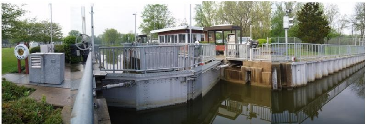
Lock - Upstream Miter Gates
