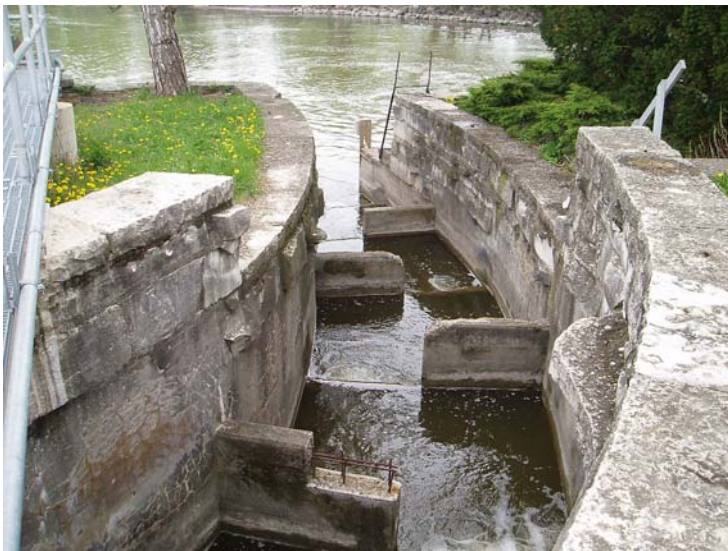
Existing Fish Ladder
