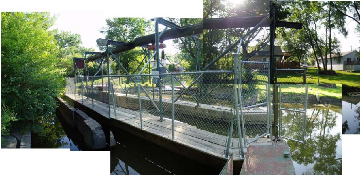
Monorail Hoist Boat Lift at Long Lake
