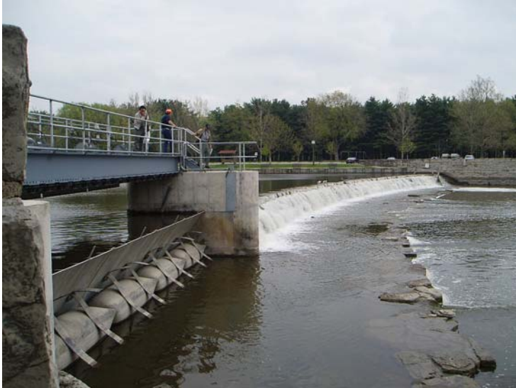
Pneumatically Operated Hinge Leaf Gate (Obermeyer)
