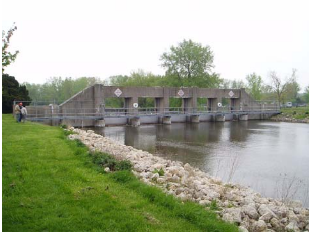
Sluice (Wheel) Gate Structure
