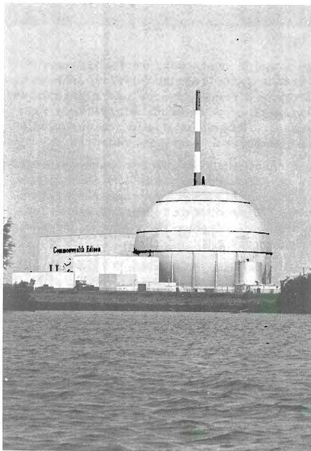
Dresden Nuclear Power Station near Morris.
