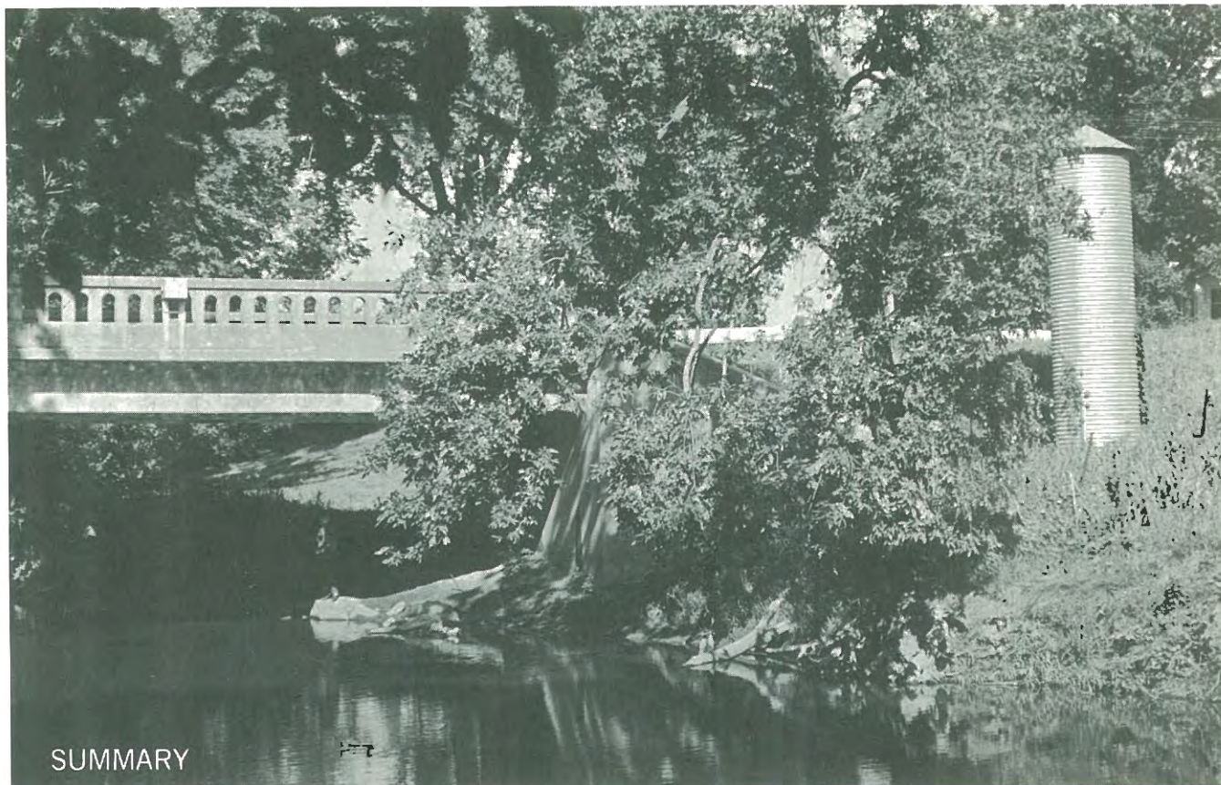
Stream gaging station.
