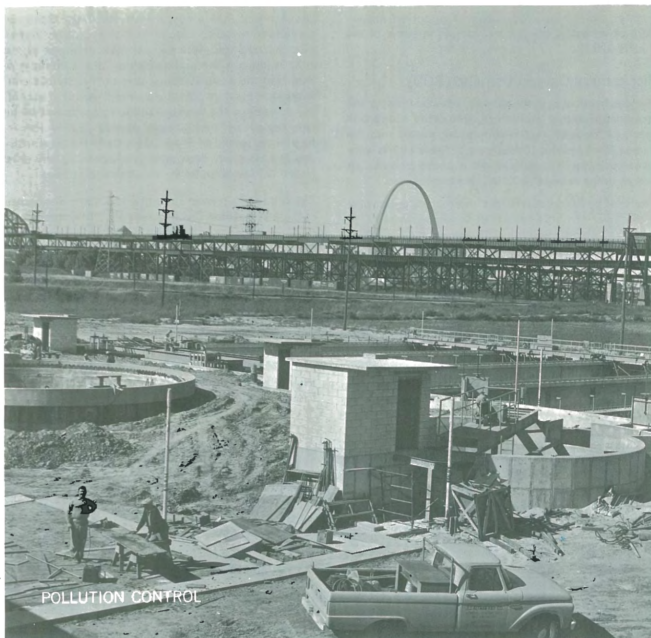
East St. Louis treatment plant under construction.
