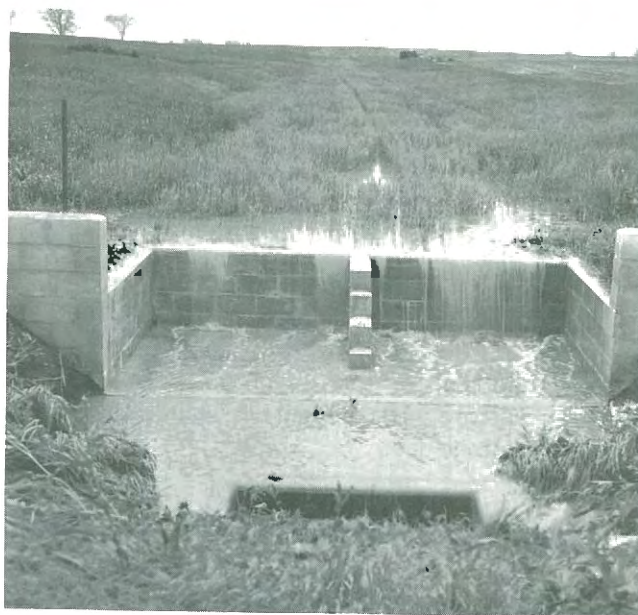
Grass waterway, Fayette County
