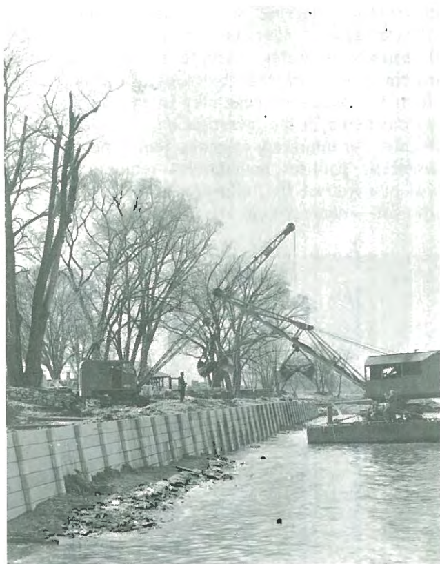
Starved Rock Seawall under construction.
